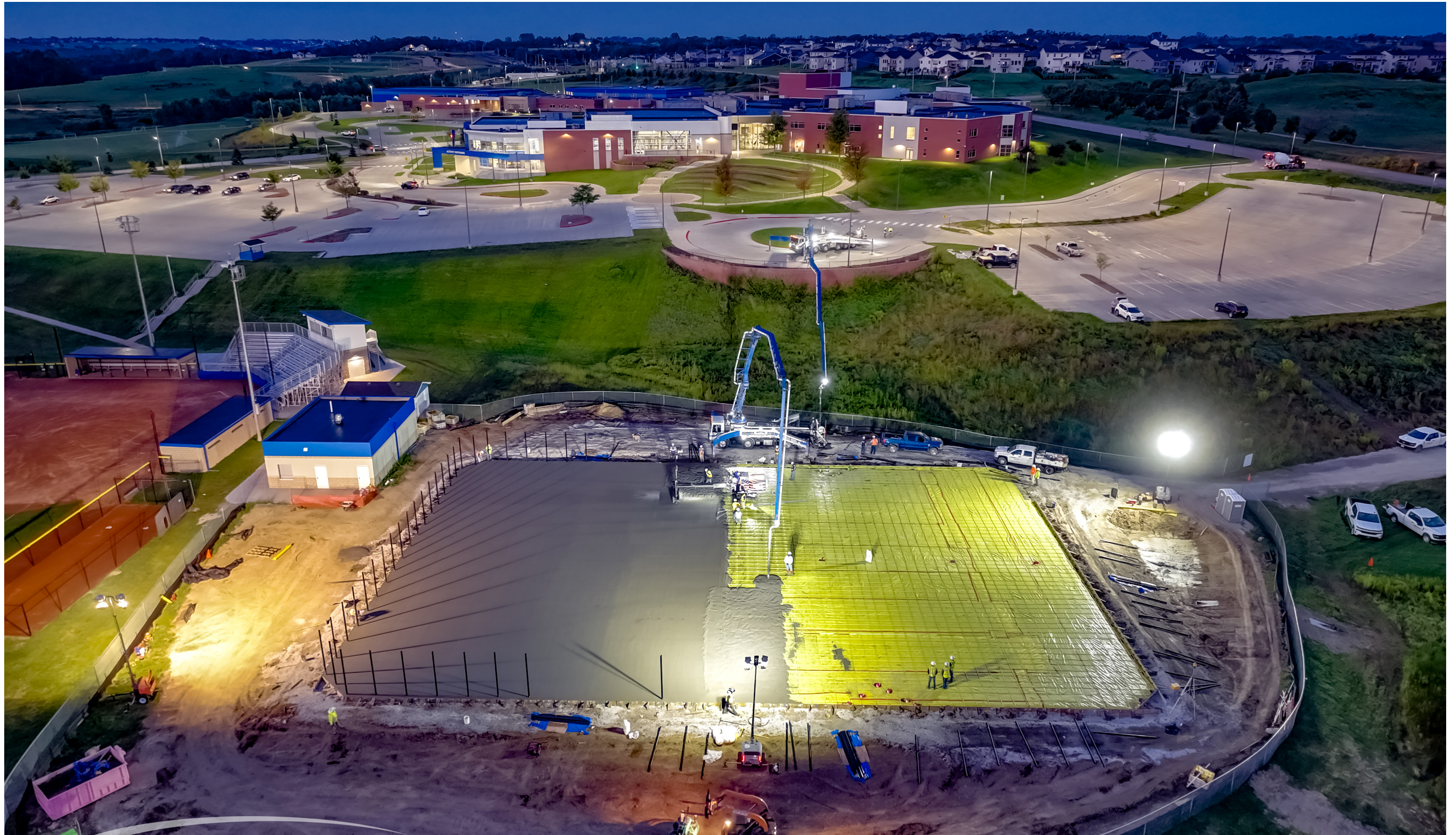
Bennington High School #2 | Tennis Court Progress 08 September 2025
