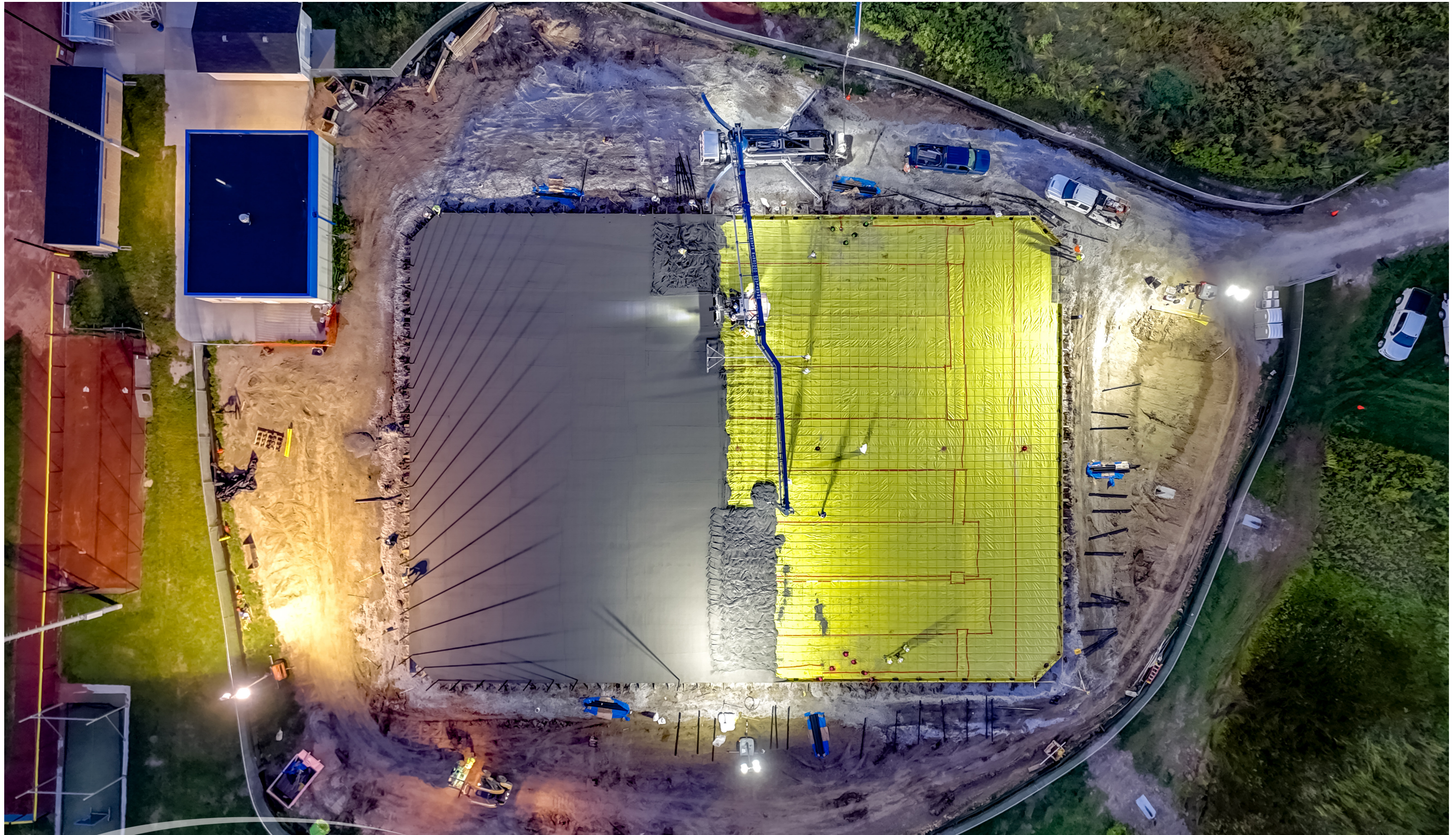
Bennington High School #2 | Tennis Court Progress 08 September 2025
