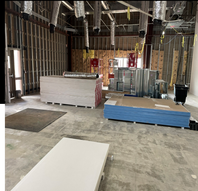
FRAMING - ROUGH-IN - DRYWALL
