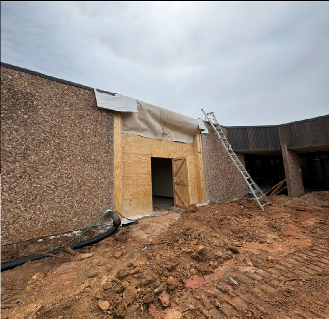
CAFETERIA TEMP PROTECTION
