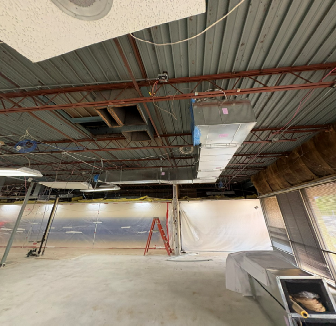
ADMIN CEILING ROUGH-IN
