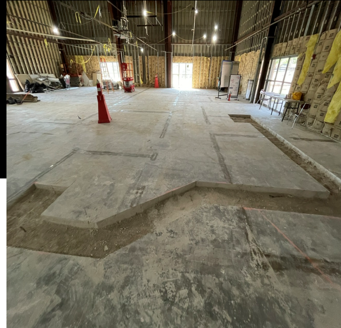
SLAB TRENCH AND WALL LAYOUT
