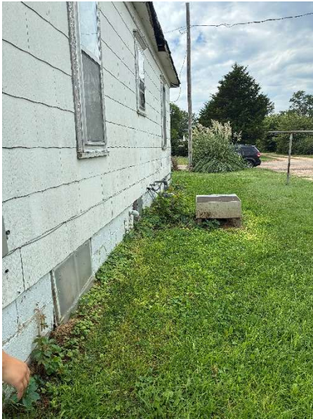
Figure Q. Vegetation conditions in north side yard
