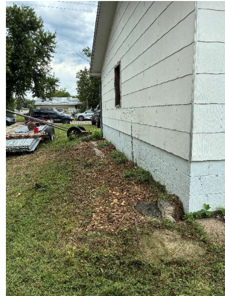
Figure R. Vegetation conditions in south side yard
