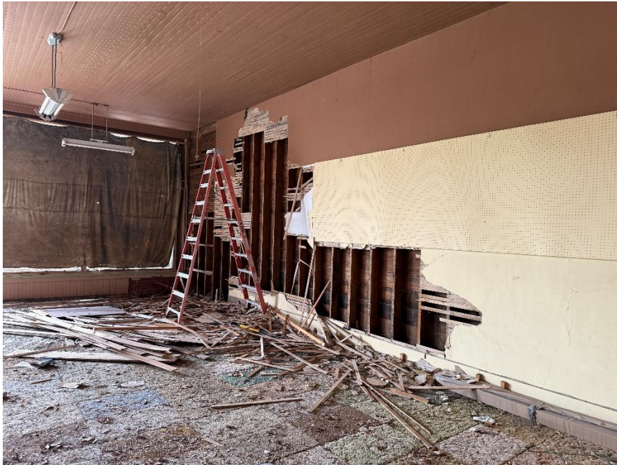
Photo 5 - East end of south first floor wall.
