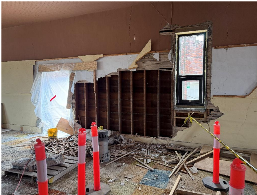
Photo 6 - South first floor wall.
