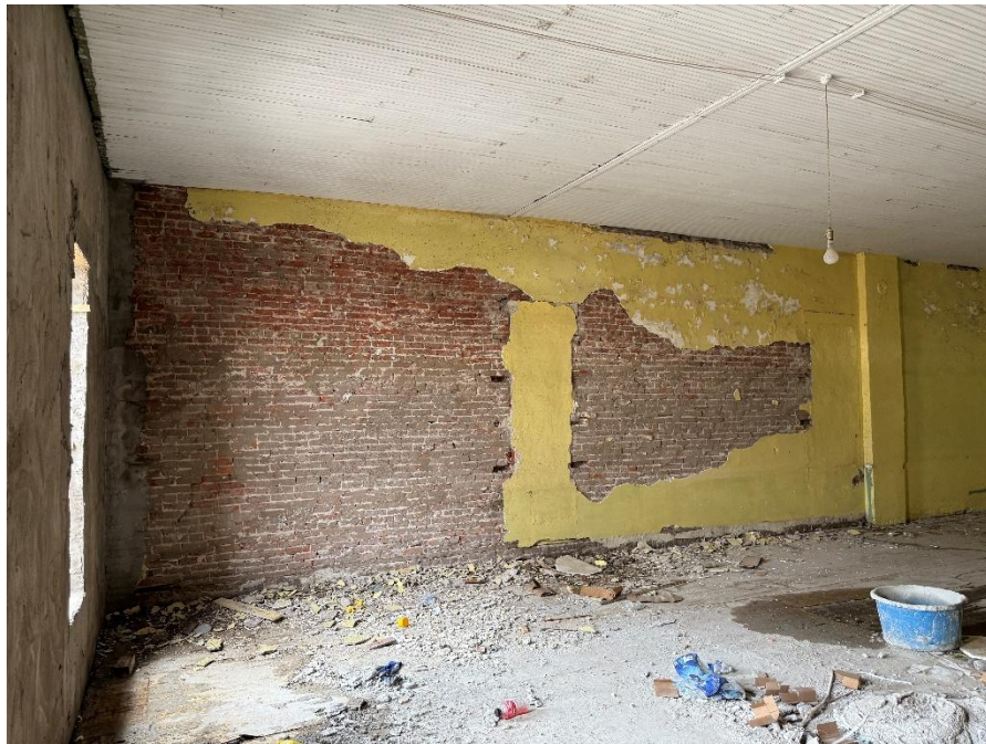
Photo 3 - Plaster removal at second floor north wall.
