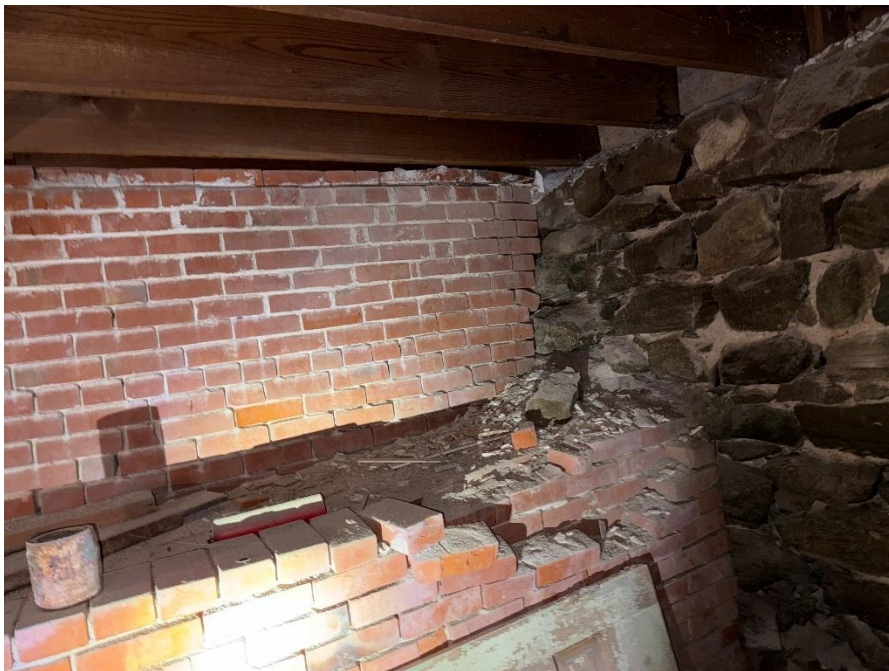
Photo 10 - Basement looking southeast.
