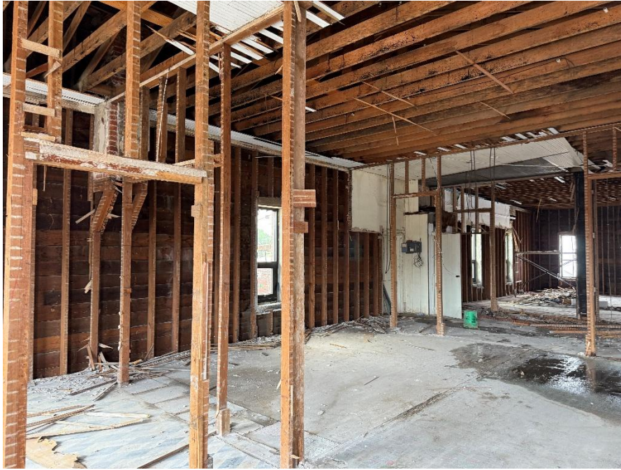
Photo 7 - Second floor wall framing.
