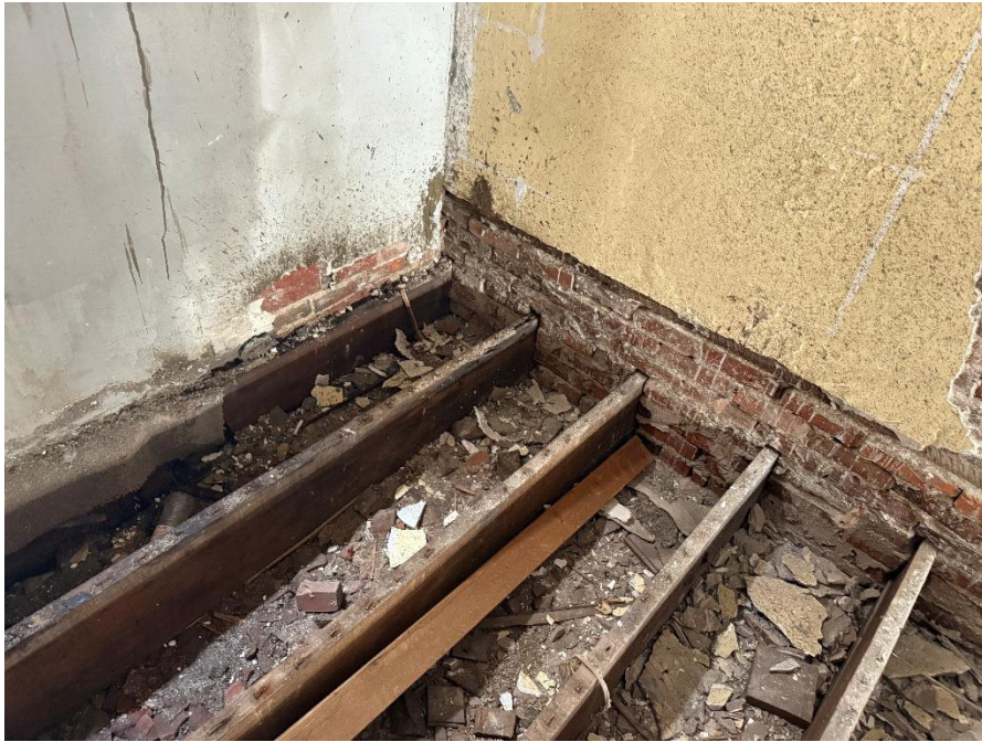
Photo 15 - Second first floor joists in from the west wall at the north building.
