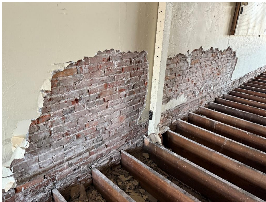
Photo 2 - Plaster removal at first floor north brick wall.
