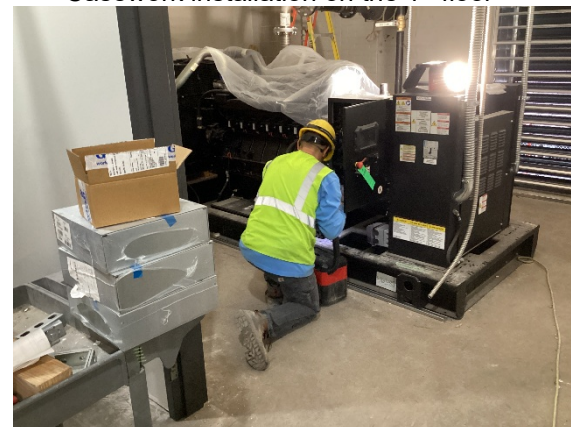
Generator rough-ins continue in the basement
