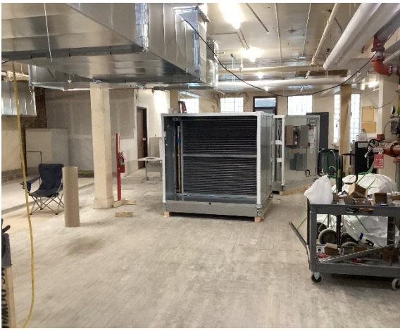
Mechanical infrastructure delivery on 3rd floor
