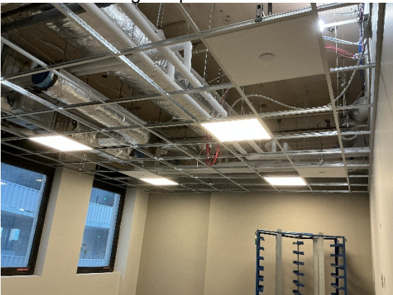
Electrical finishes on the 1 st floor
