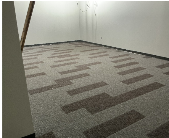
Flooring installation on the 1 st floor
