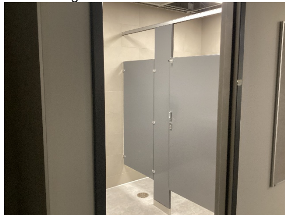
Bathroom partitions on the 2 nd floor
