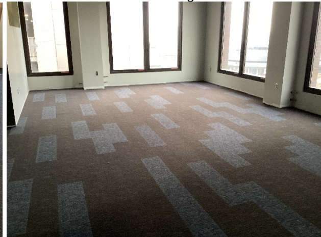
2nd Floor Carpet Installation
