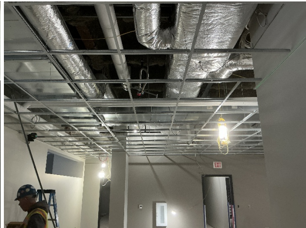
2nd Floor Ceiling Grid Installation
