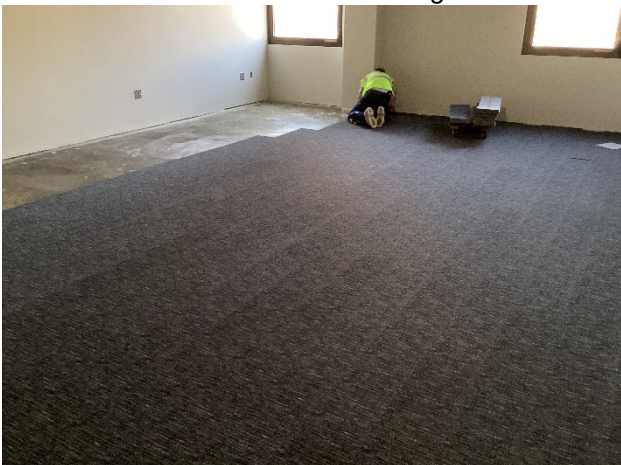
2nd Floor Carpet Installation
