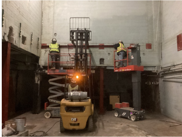
Structural Steel Erection
