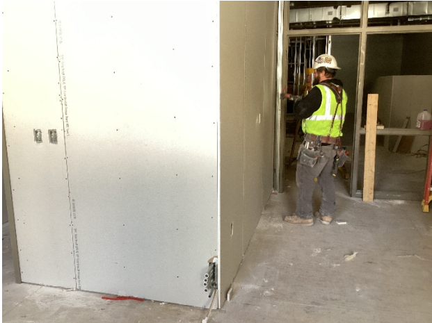
Drywall Installation
