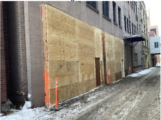
Exterior Wall Temporary Enclosure
