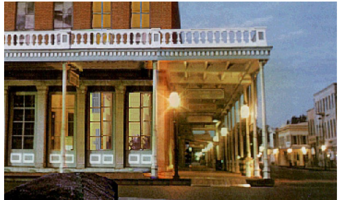
A GALLERY WITH SLENDER METAL COLUMNS.
