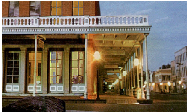
A GALLERY WITH SLENDER METAL COLUMNS.
