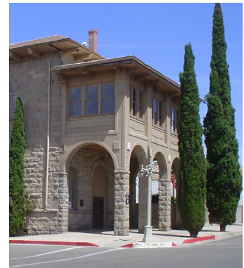
A MASONRY GALLERY WITH HABITABLE SPACE ON THE SECOND FLOOR.
