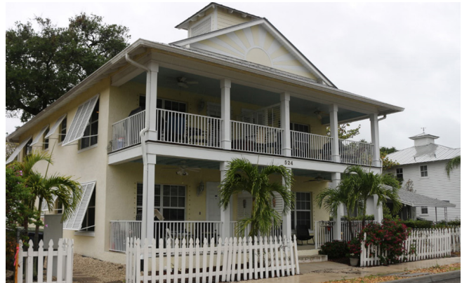
A 2-STORY PORCH ON AN APARTMENT BUILDING.
