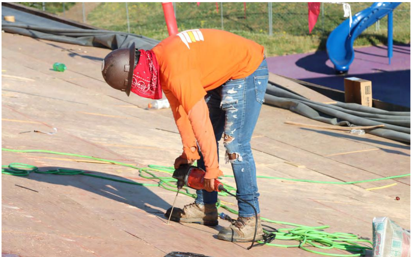
Reike Elementary Roof Project, July 26, 2022
