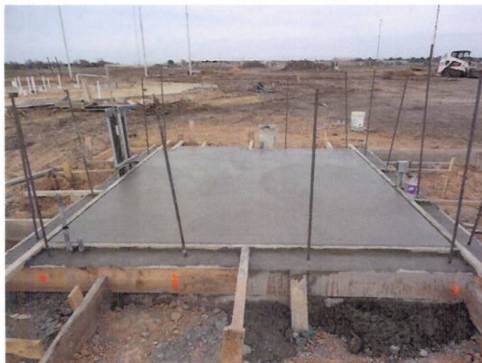
5. Ticket booth concrete foundation
