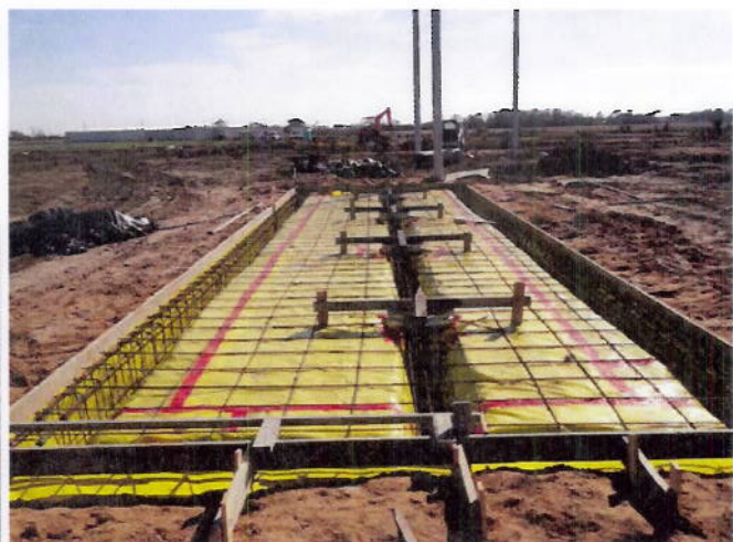
6. Softball Field: 1 st base dugout foundation prep.
