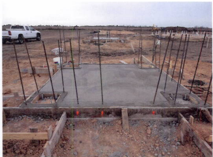
4. Entry pavilion concrete foundation
