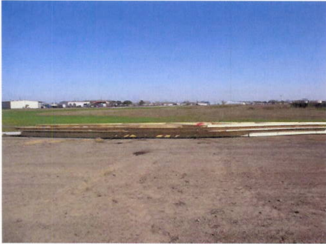
1. Wood truss delivery / Concession and Front Entry
