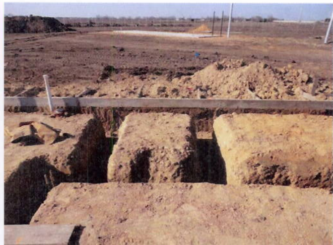
10. Concession stand grade beam excavation
