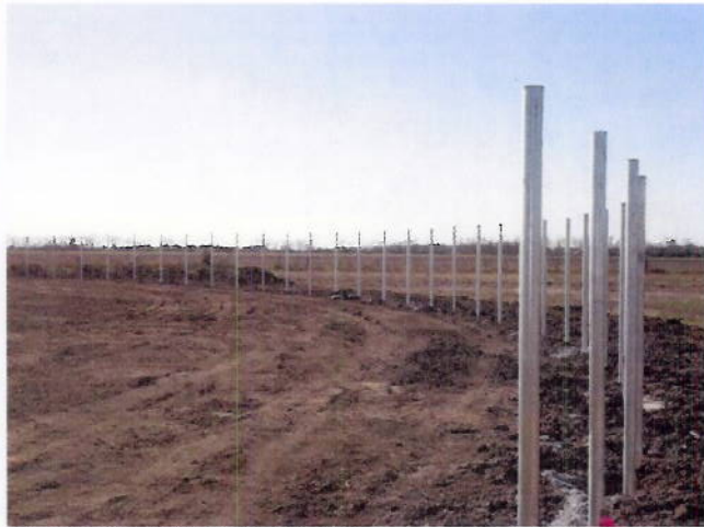
4. Softball Field: Outfield fence post installation
