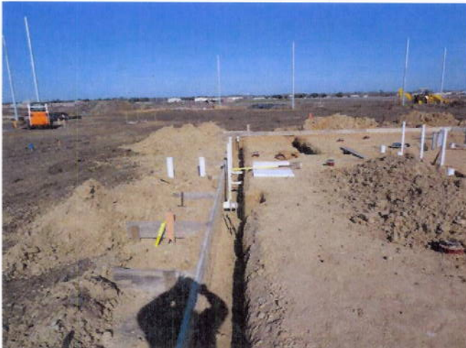
9. Concession stand grade beam excavation
