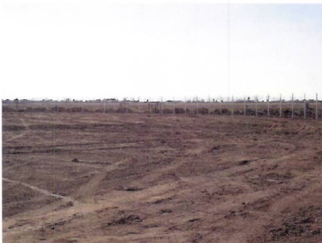
5. Softball Field: Outfield fence post installation
