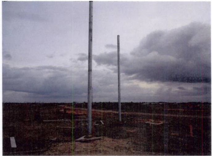
2. Softball field backstop netting supports
