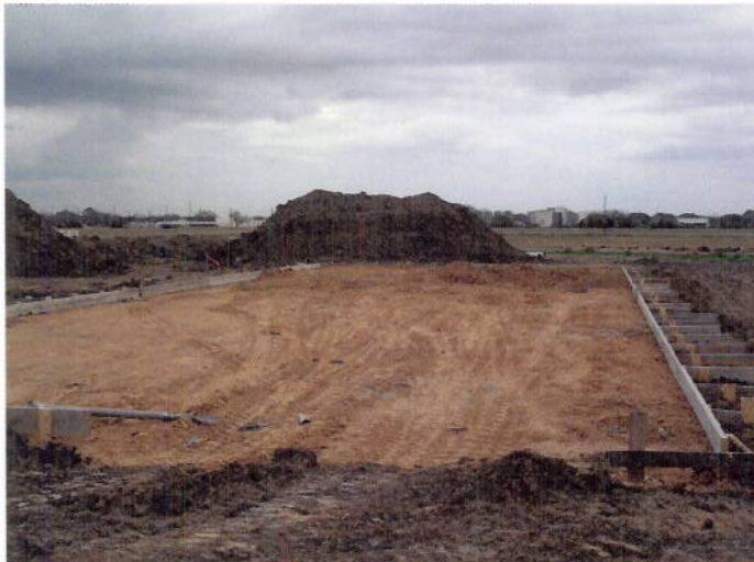
3. Baseball batting cage concrete formwork
