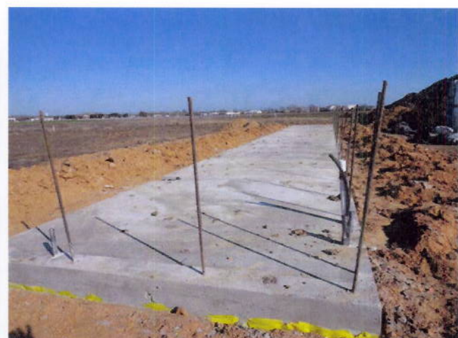
12. Baseball: 1 st base dugout foundation
