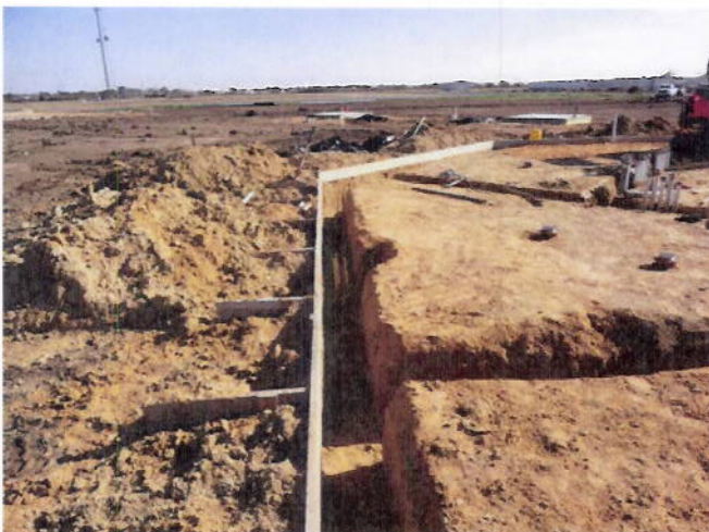
11. Concession stand grade beam excavation
