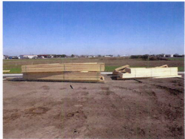
2. Wood truss delivery / Concession and Front Entry
