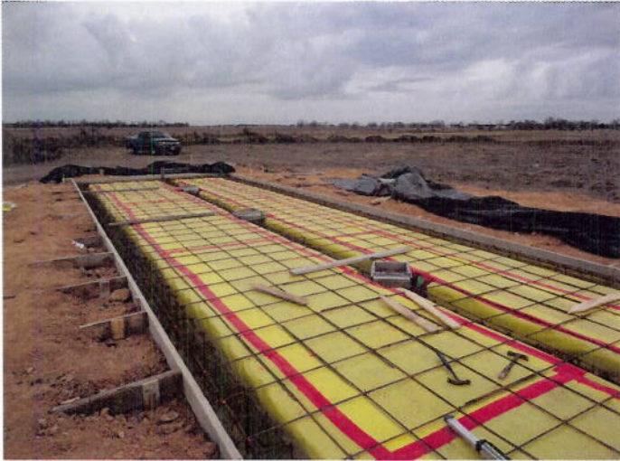
1. Foundation preparation at Softball Dugout
