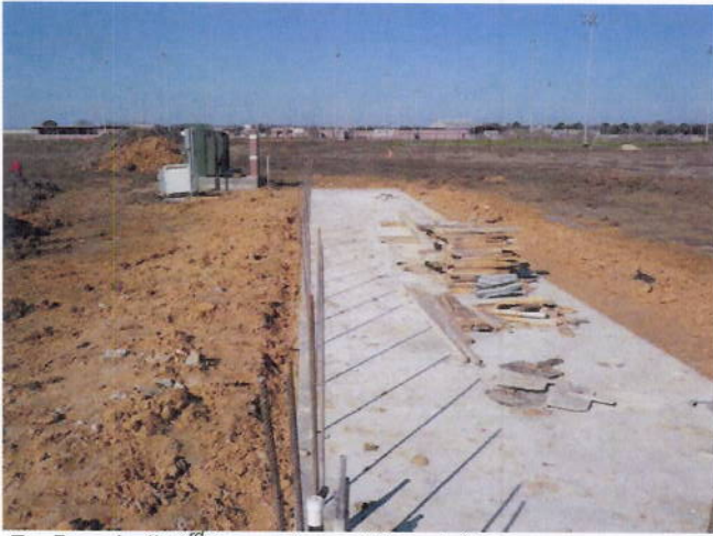
7. Baseball: 3 rd base dugout foundation
