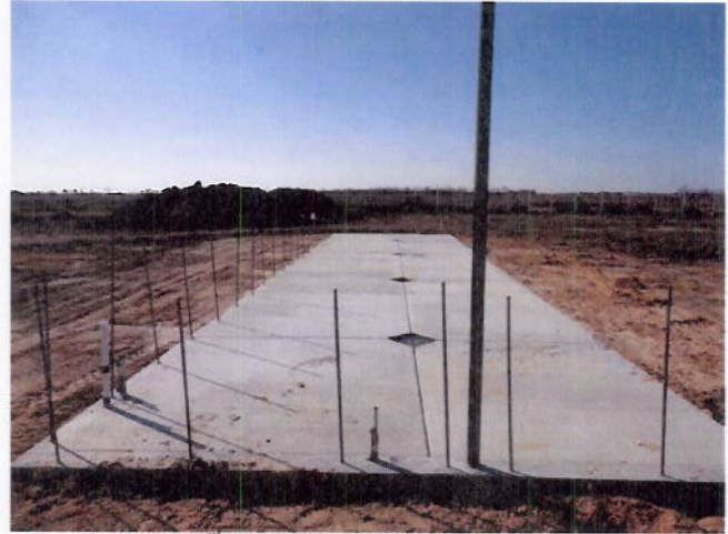
8. Softball: 3 rd base dugout foundation
