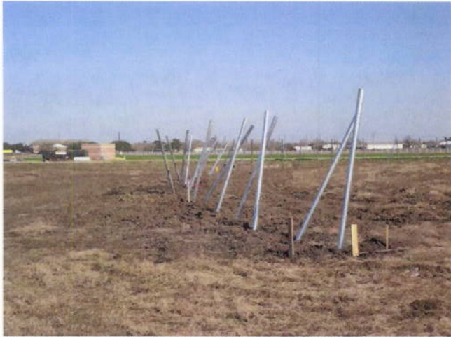
3. Baseball Field: Outfield fence post installation
