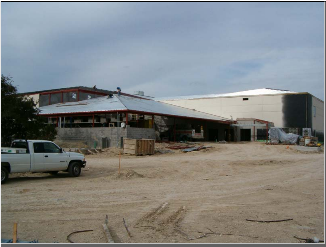
South East Corner of the building, Kitchen / Cafeteria - December 2004
