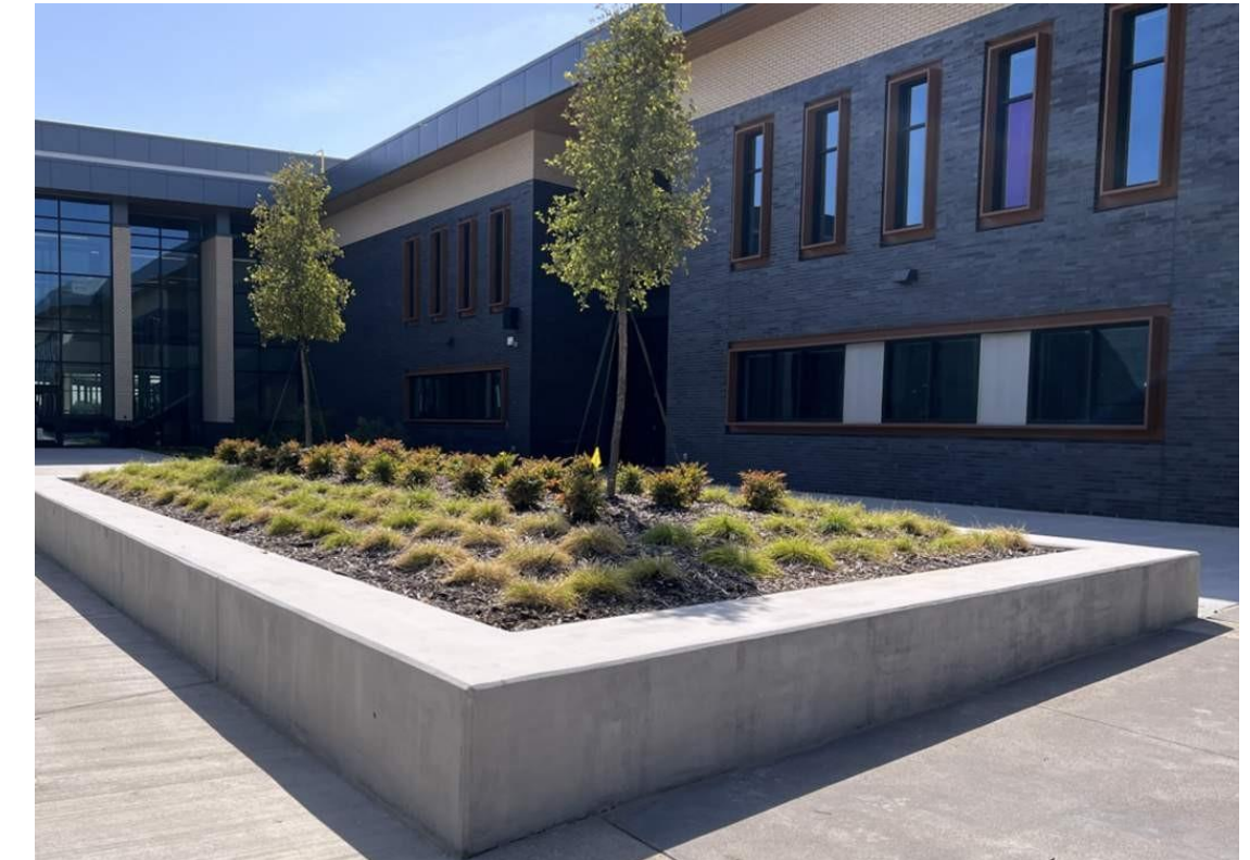
Concrete Seat Wall Planter
