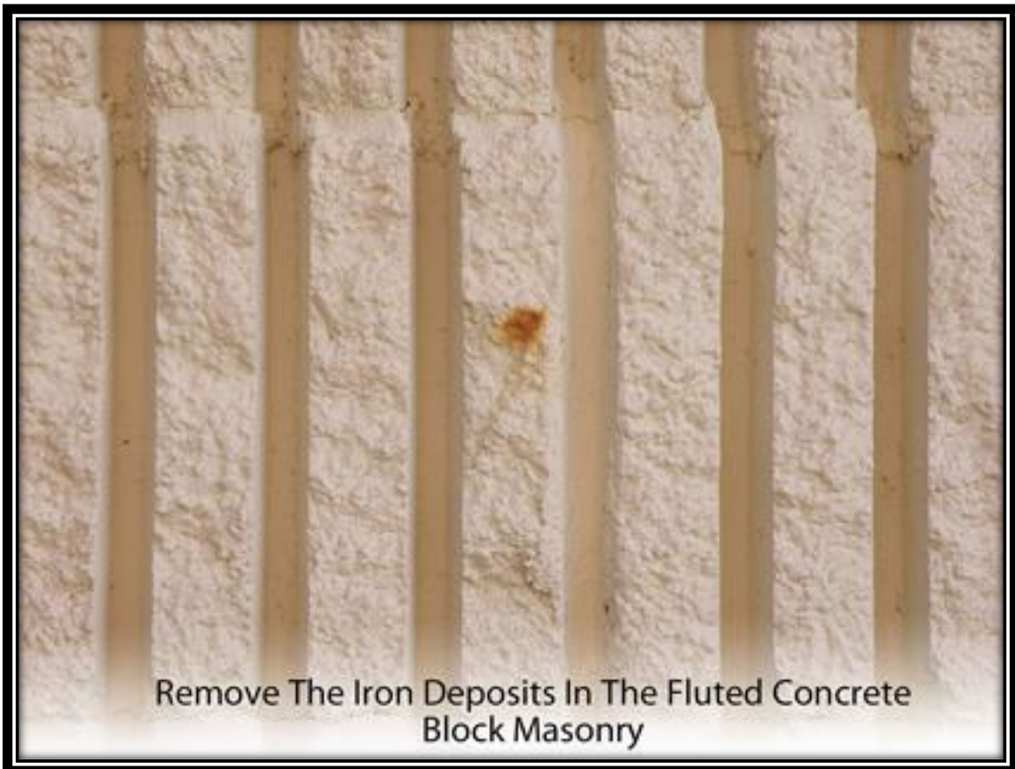
Remove The Iron Deposits In The Fluted Concrete Block Masonry
