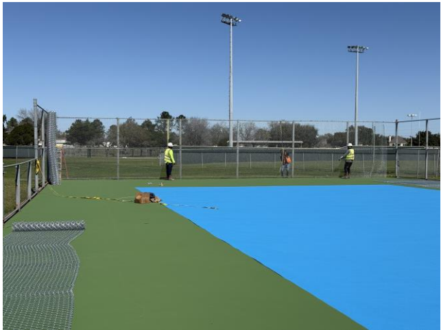
Installing Fence at Court 11 & 12
