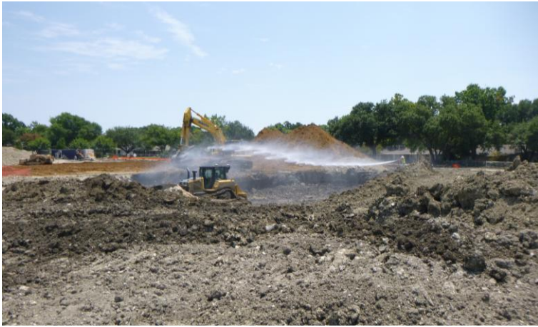
(Above) Ongoing soil conditioning on site | (Below) Fire lane complete
