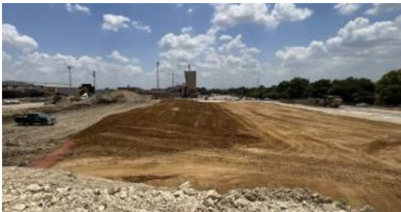
(Above) Moisture conditioning of site | (Below) Southwest aerial view of site at Dogwood
