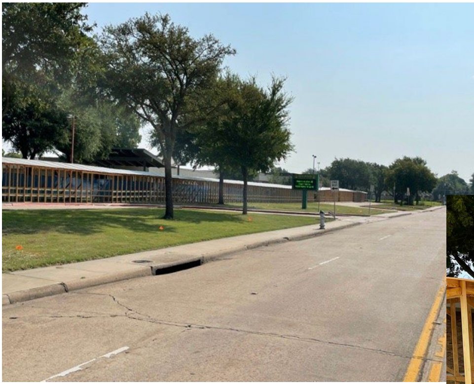
Temporary walkway between buildings
