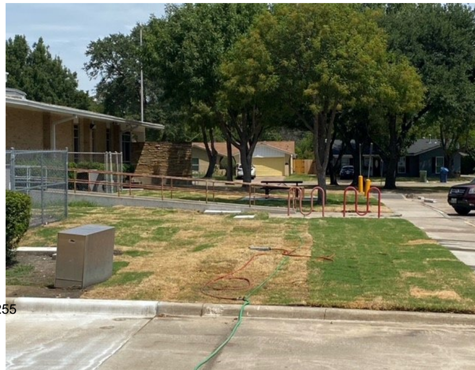
O Henry ES - Sewer Line Replacement
