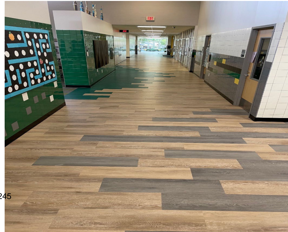
Dartmouth ES – New LVT in Corridor
