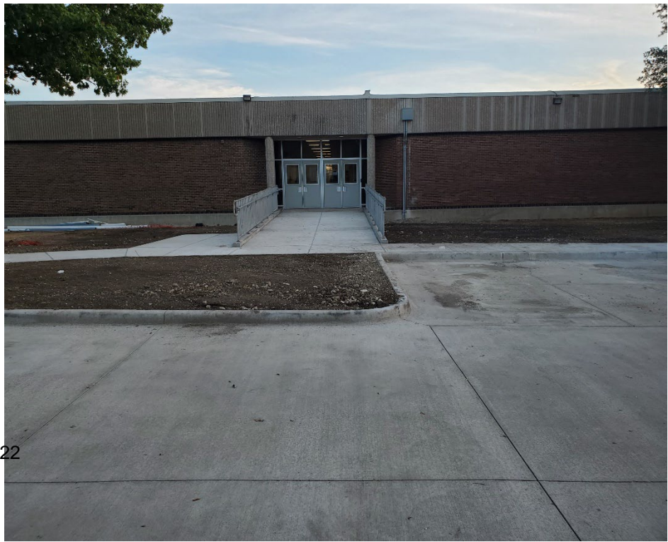
Temporary Front Main Entry
