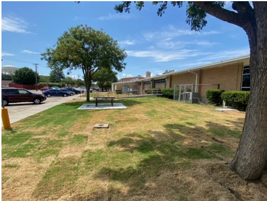
O Henry ES - Sewer Line Replacement
