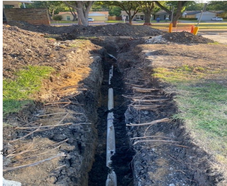
O Henry ES - Sewer Line Replacement
