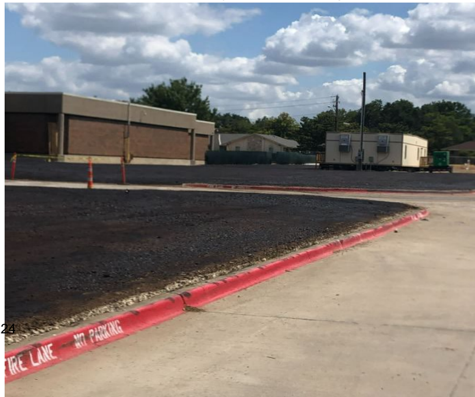
Temporary Staff Parking
