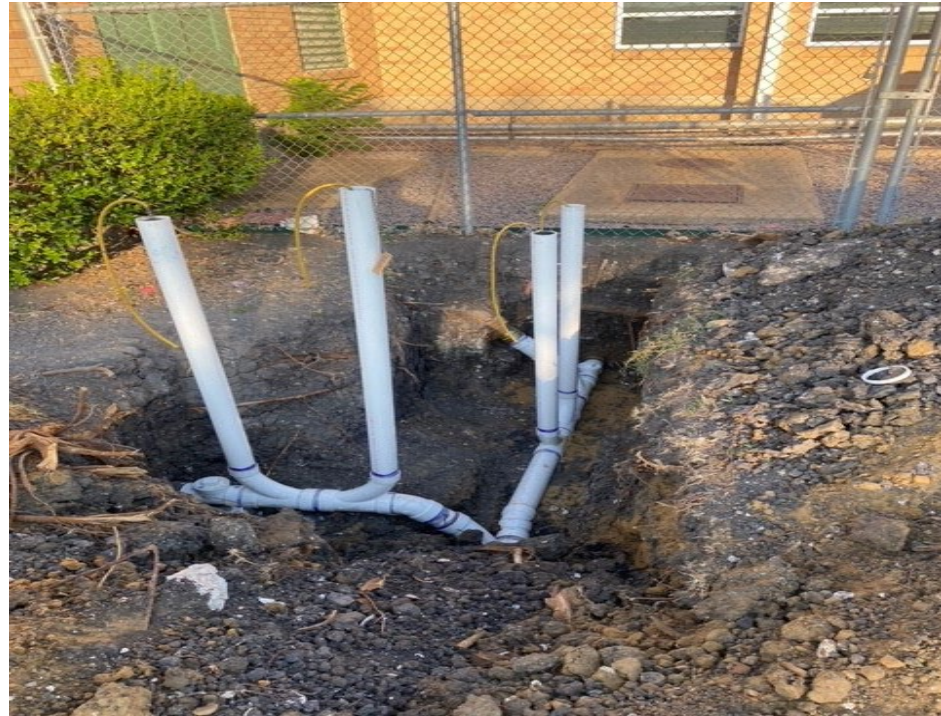
O Henry ES - Sewer Line Replacement
