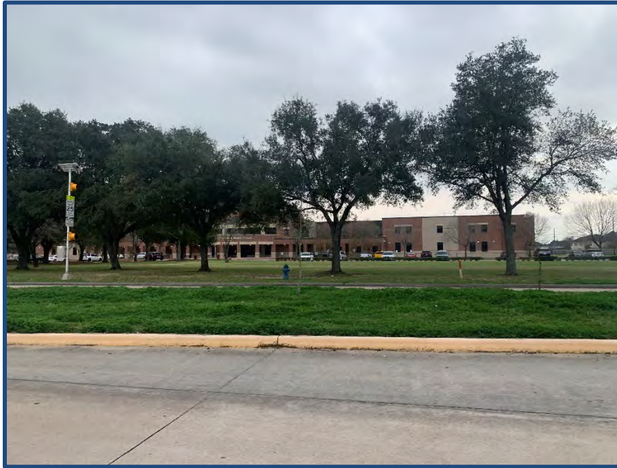
View of subject facing main improvements (not impacted)
