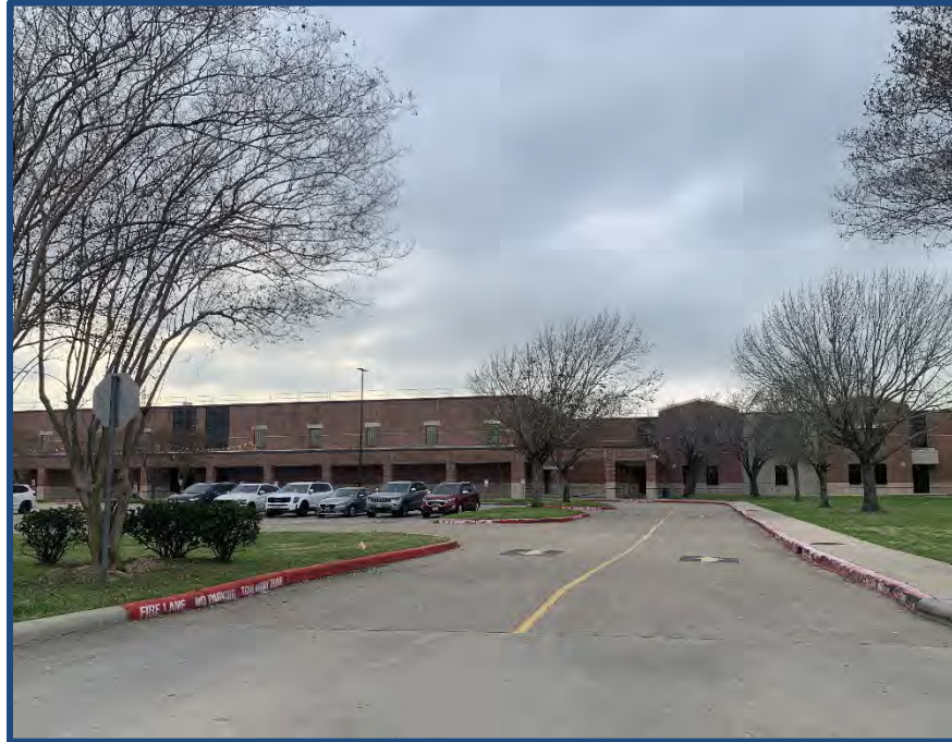
View of north entrance to subject from Barker Cypress Road
