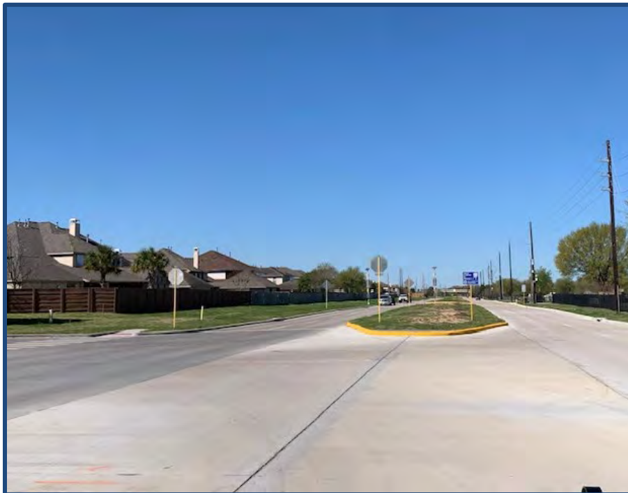
View west along Schiel Road at intersection with Fairfield Place Drive
