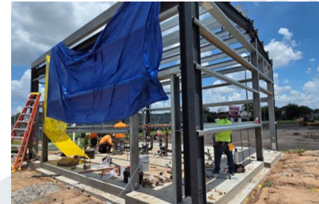
Dulles HS BB/SB Restroom
