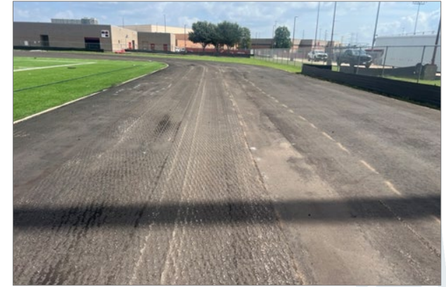
Travis HS Track Resurfacing
