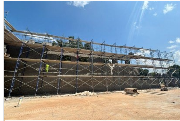
Palmer ES Gym Addition
