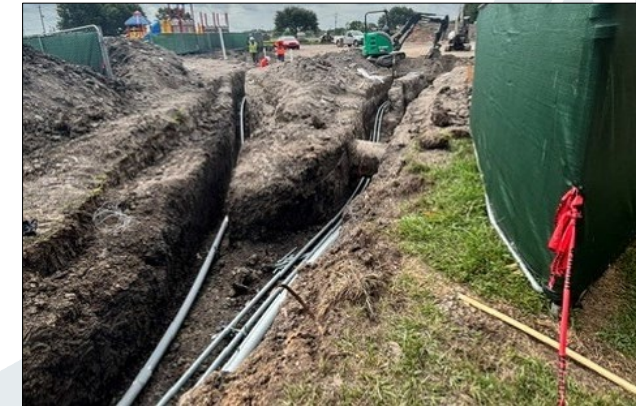
Hunters Glen ES Gym Addition
