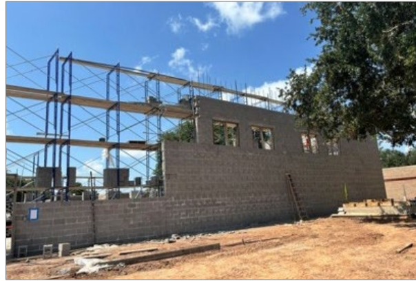
Palmer ES Gym Addition
