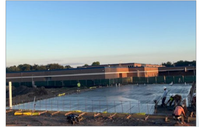
Hunters Glen ES Gym Addition
