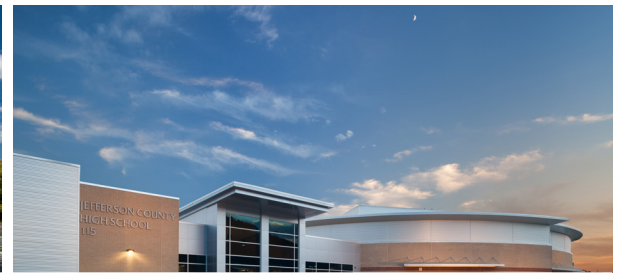
JEFFERSON COUNTY HIGH SCHOOL
