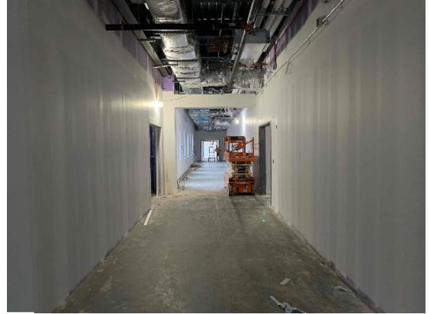
PAC Main Corridor - 1st Coat Paint
