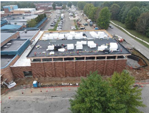
Gym North Elevation - Brick Veneer 90% Complete
