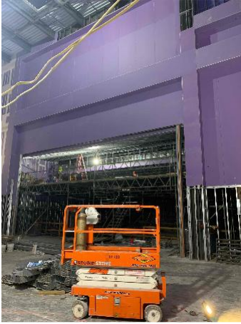
PAC Stage - Hang and Finish Drywall
