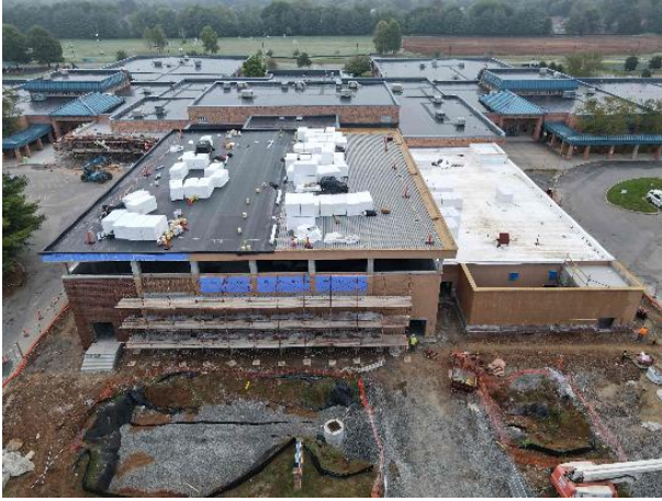
Gym West Elevation - Exterior Brick
