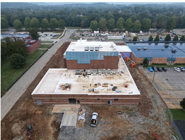
East Elevation- Insulated Metal Panels 100% Complete
