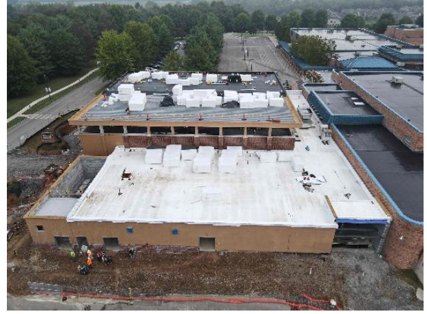
Gym South Elevation - High Roof - 50% Complete
