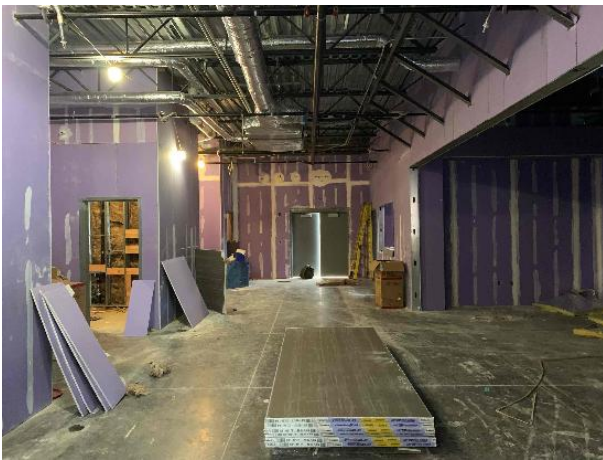
PAC Legacy Gallery - Hang and Finish Drywall
