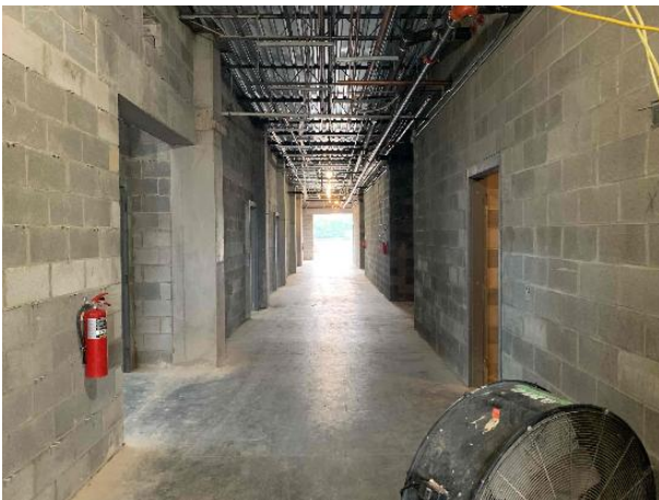
Gym Main Hallway - Above Ceiling - Mechanical Electrical and Plumbing
