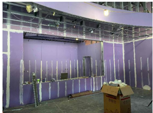
PAC Concession Stand - Hang and Finish Drywall
