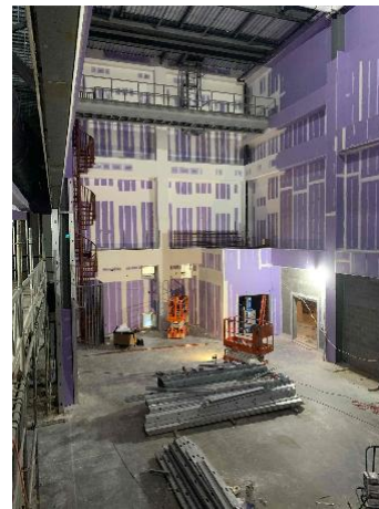
PAC Stage - Hang and Finish Drywall
