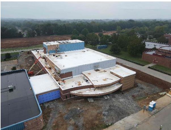
West Elevation- Insulated Metal Panels 80% Complete
