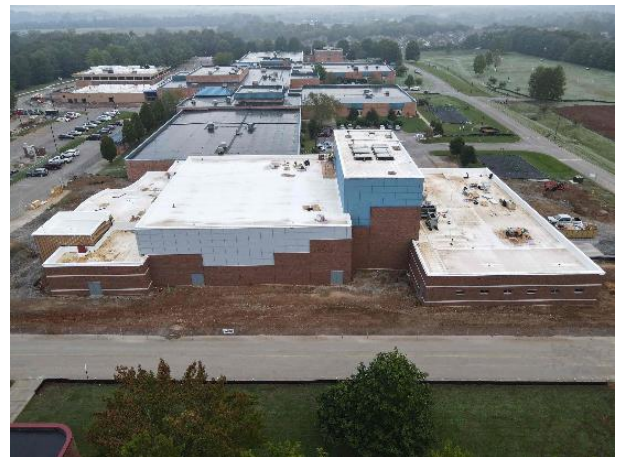
South Elevation- Insulated Metal Panels 100% Complete
