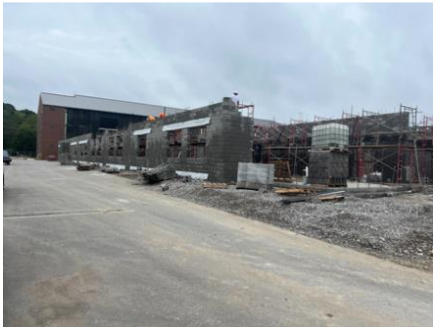
Area C CMU Block Installation
