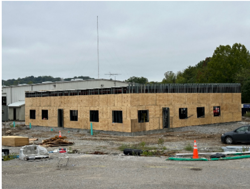
Building with Wall Sheeting
