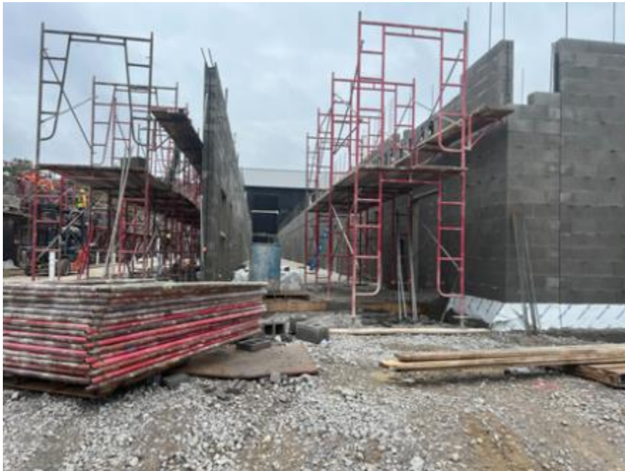
First Floor Corridor
