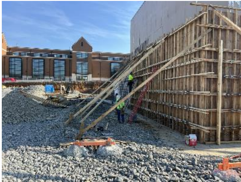
Retaining Wall Forms
