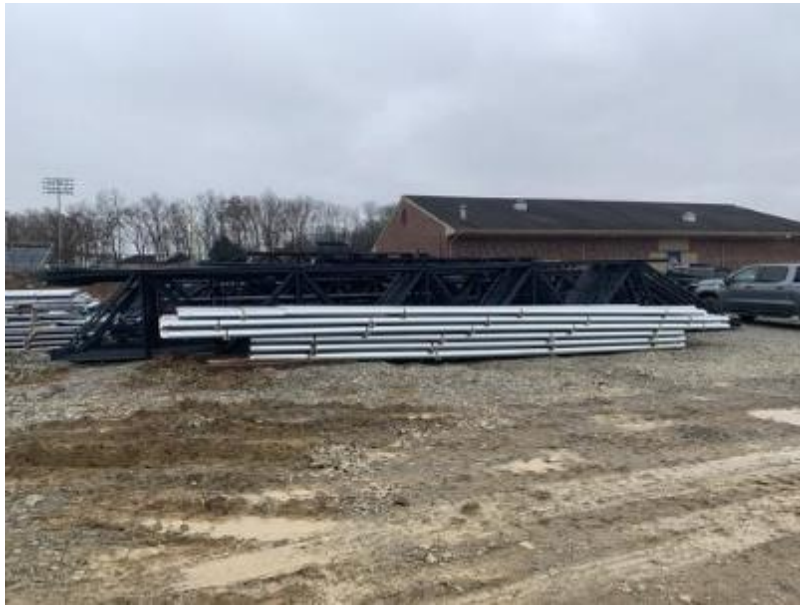
Roof System Trusses
