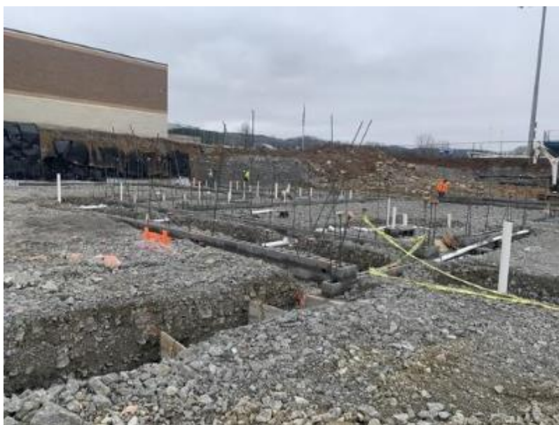
Footings and Foundation Walls
