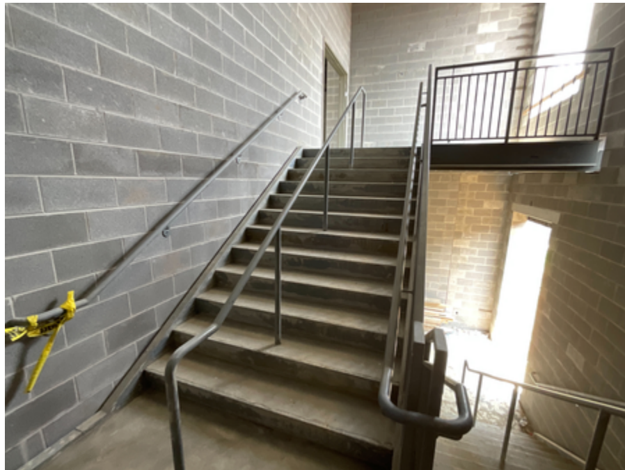
Stairwell to Third Floor
