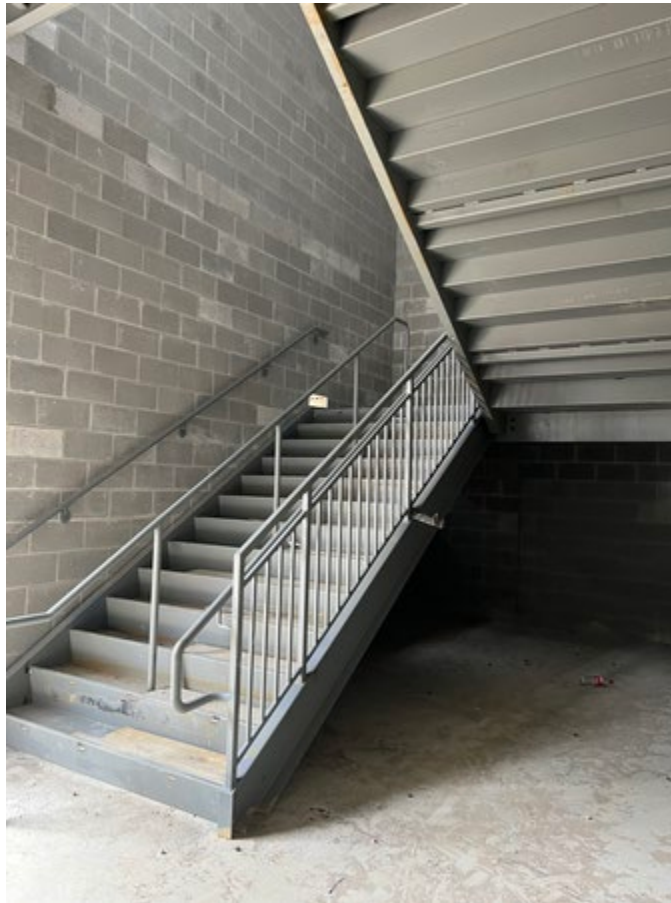
Area A Stairs
