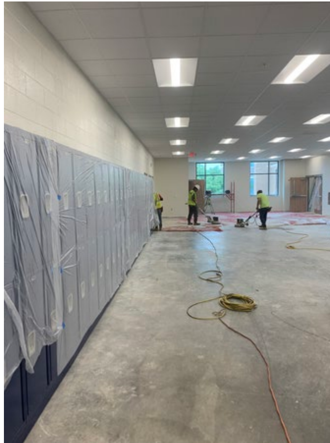
Lockers and floor prep
