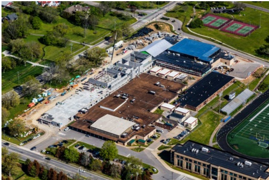
Aerial view of progress
