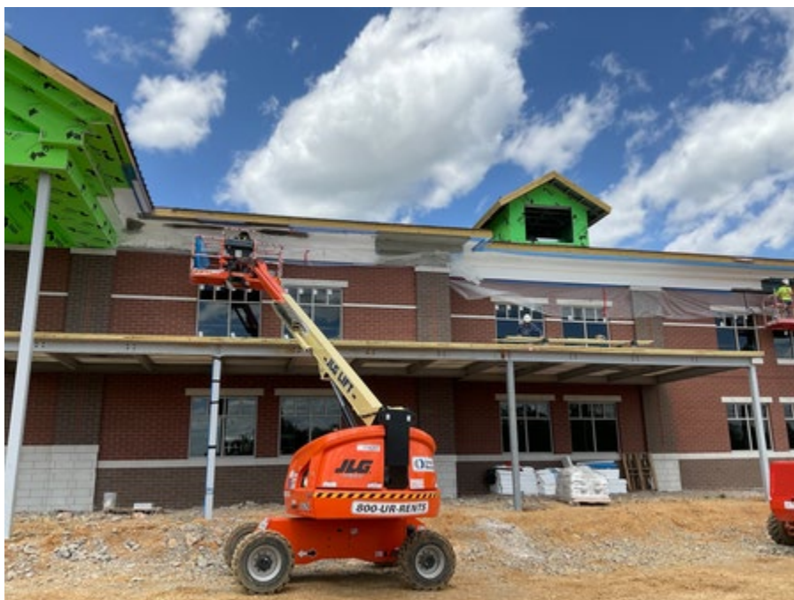
Front of Building
