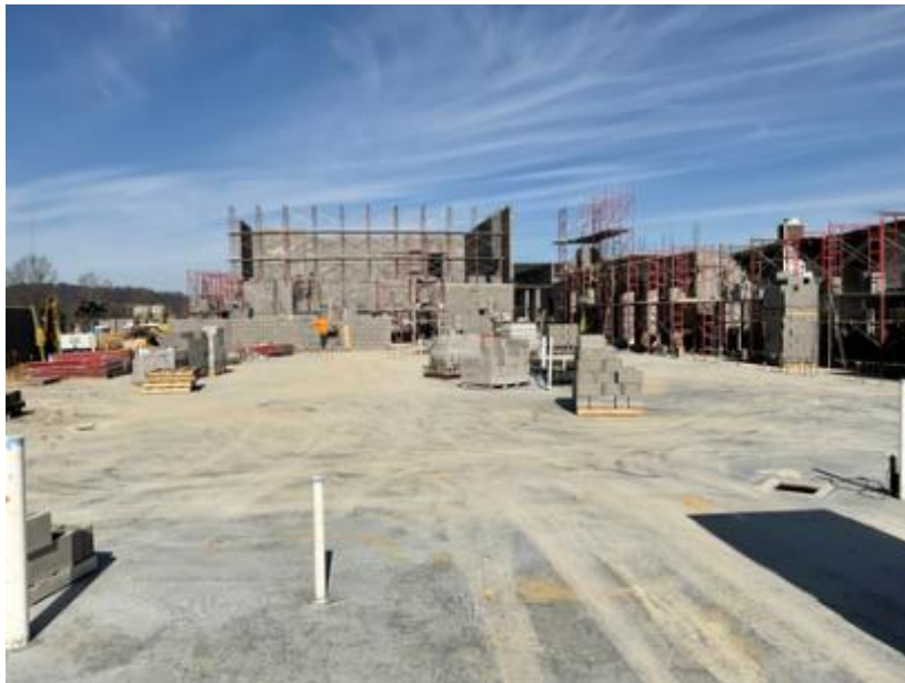
Auditorium walls and A wing slab
