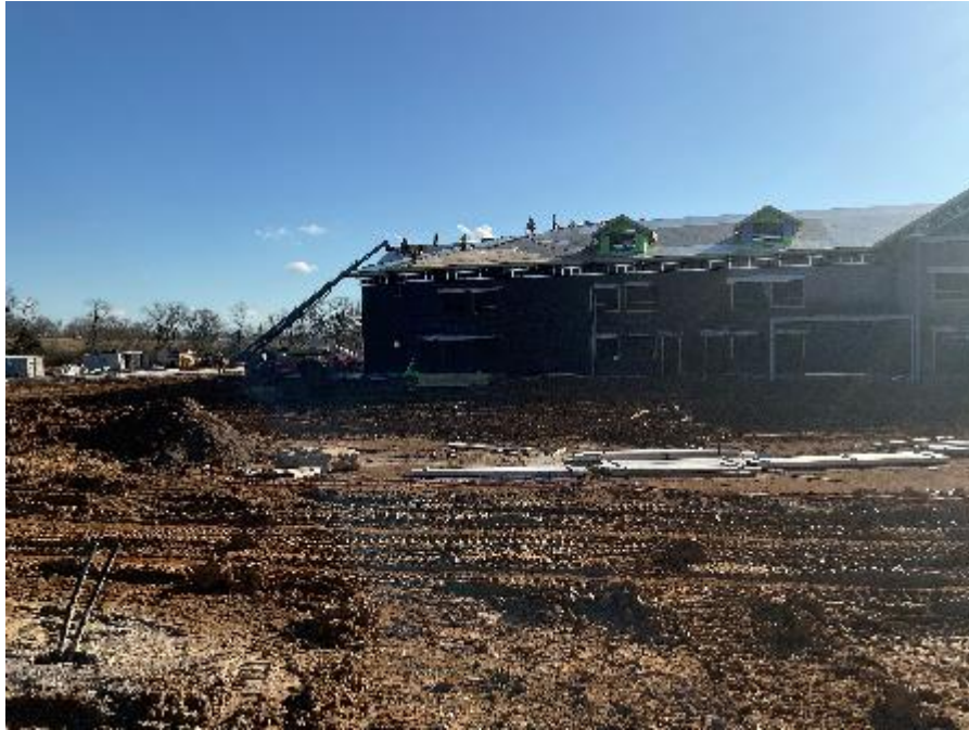
F Wing Roofing
