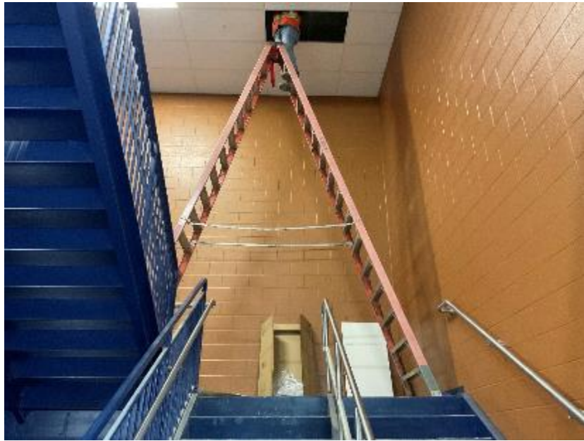
Stairwell Light Installation
