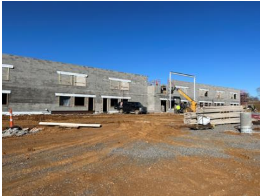
Rear of building
