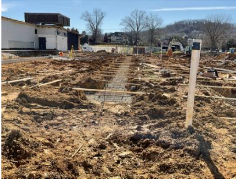
B wing Footings
