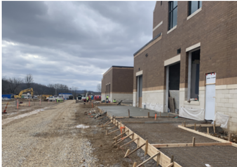
Sidewalks on the east side of building
