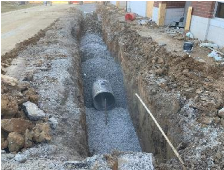
Storm Sewer Installation
