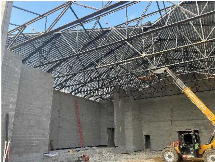
Gymnasium Roof Installation
