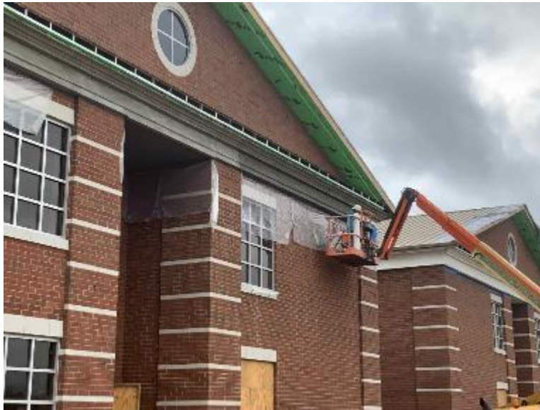
Roofing, Eaves, and Gutter
