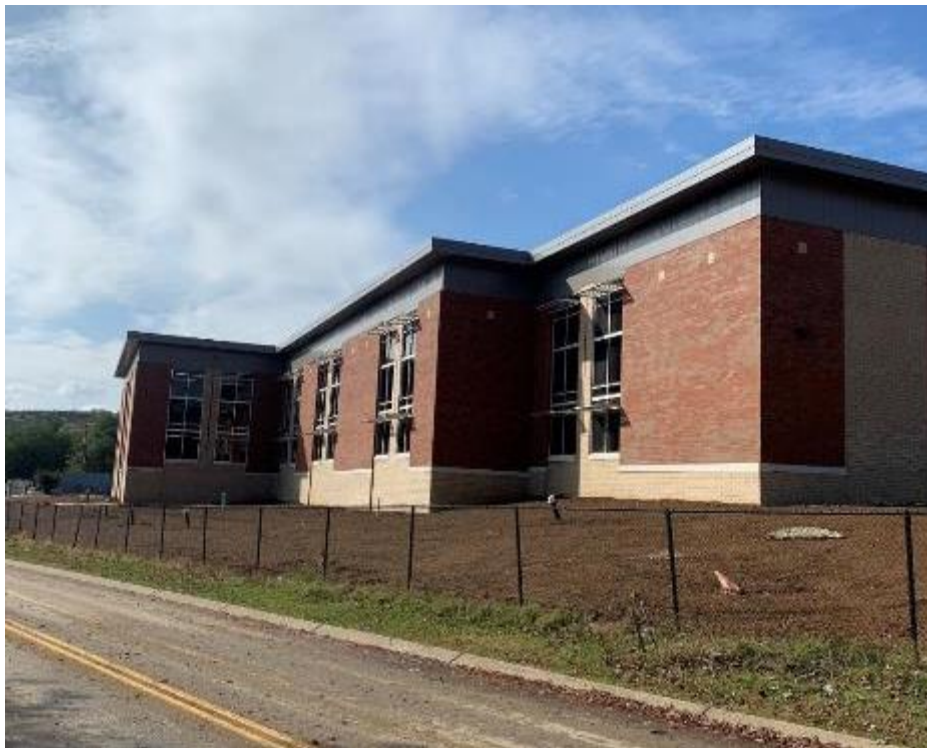
Final Exterior Complete, Site Prepped for Sod
