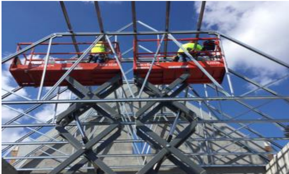
Metal Truss Installation
