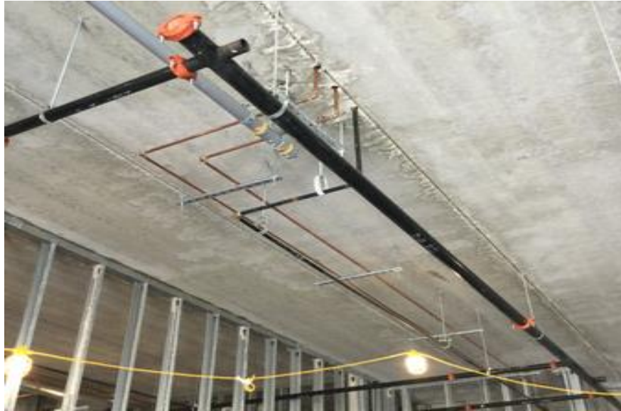
Roof over kitchen
