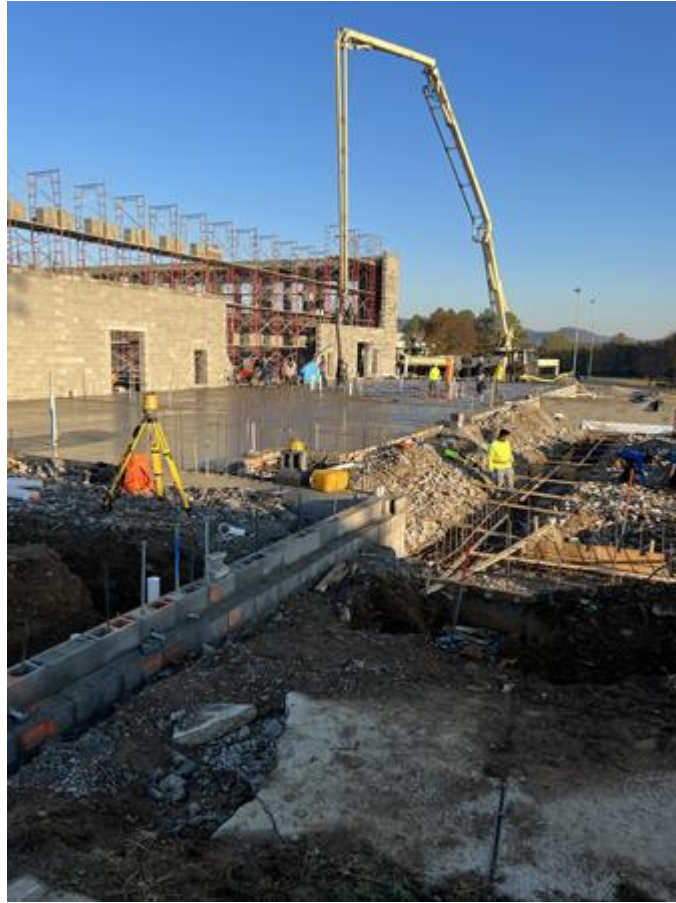
Area D Locker rooms
