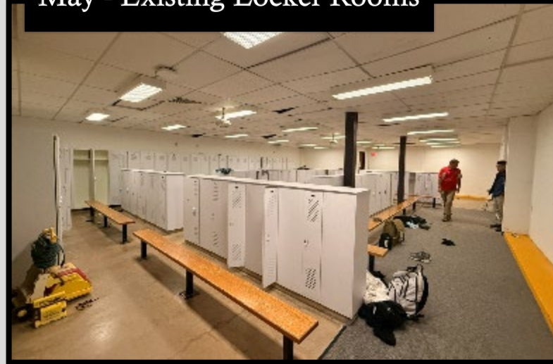
May - Existing Locker Rooms
