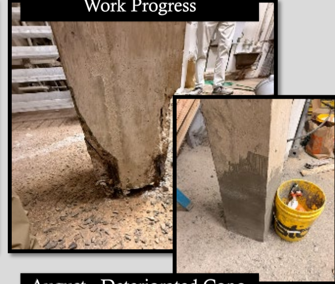
August - Deteriorated Conc. Work Progress
