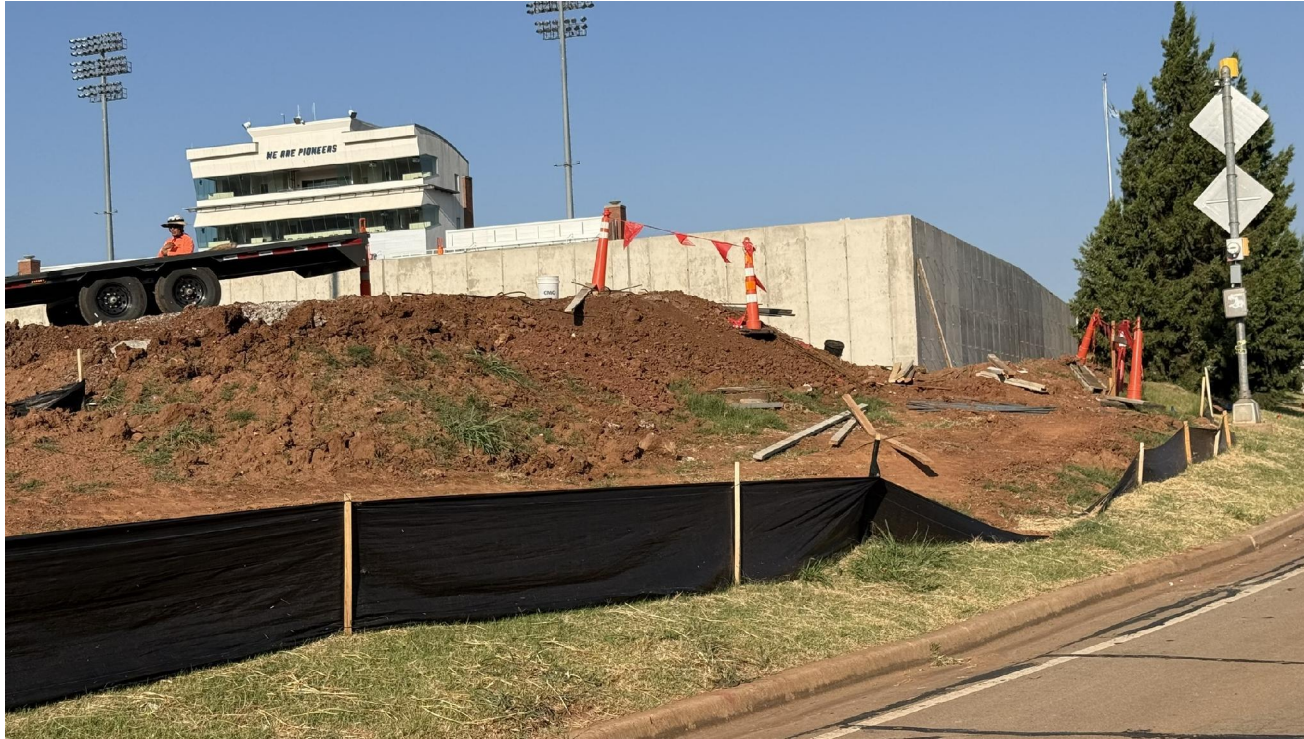
NORTH RETAINING WALL AT POLE VAULT
