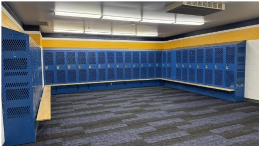
FIELD HOUSE LOCKER ROOMS RENOVATION
