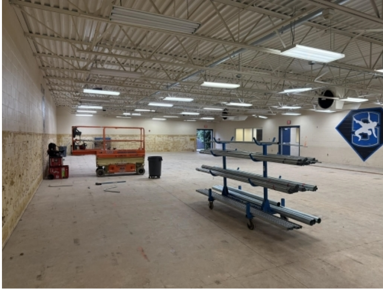
INDOOR DEMOLITION OF THE FUTURE SOCCER, TRACK AND XC BUILDING
