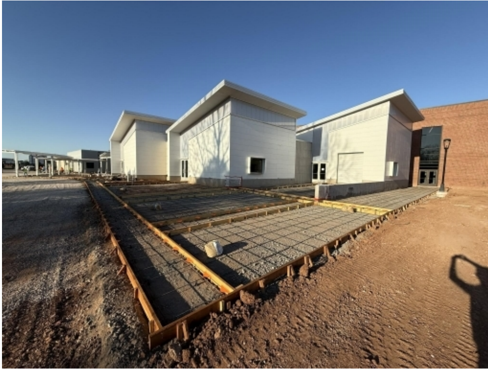
EXTERIOR – VISUAL ARTS PLAZA AREA
