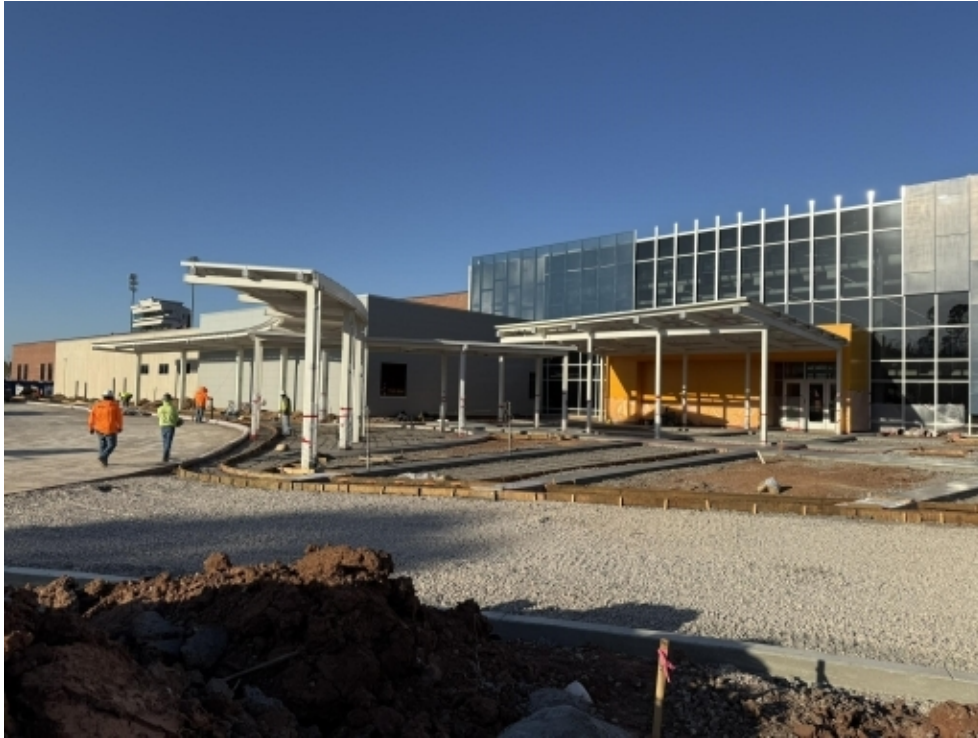
EXTERIOR – BUS DROP-OFF / PIONEER PLAZA / SECONDARY ENTRY PAVING
