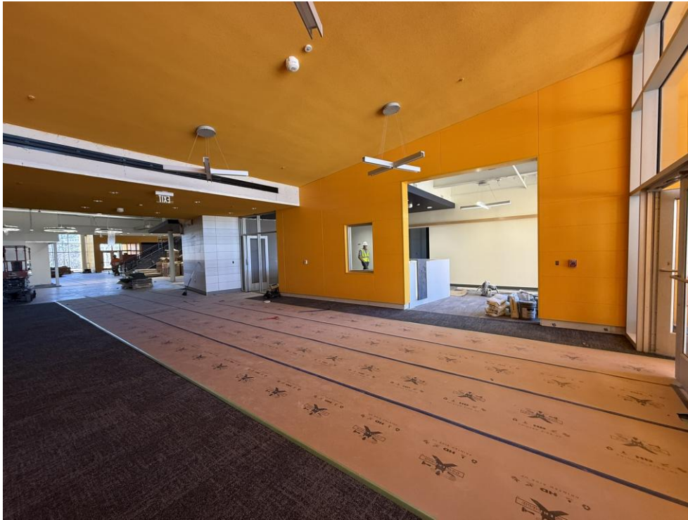
FRONT ENTRY SECURE LOBBY AREA
