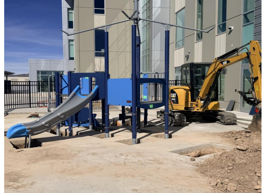
Preschool playground equipment installed
