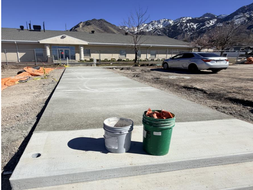
Sidewalk to Seminary Building is complete
