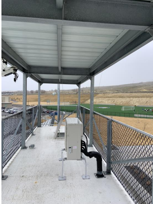
Grandstands heat 19 pump installation
