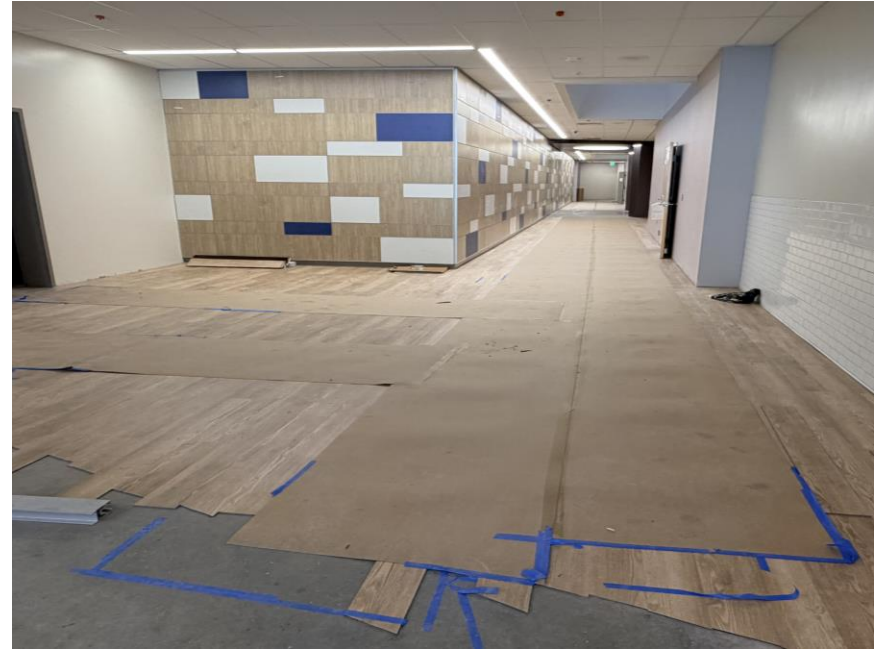
Corridor LVT being installed and protected
