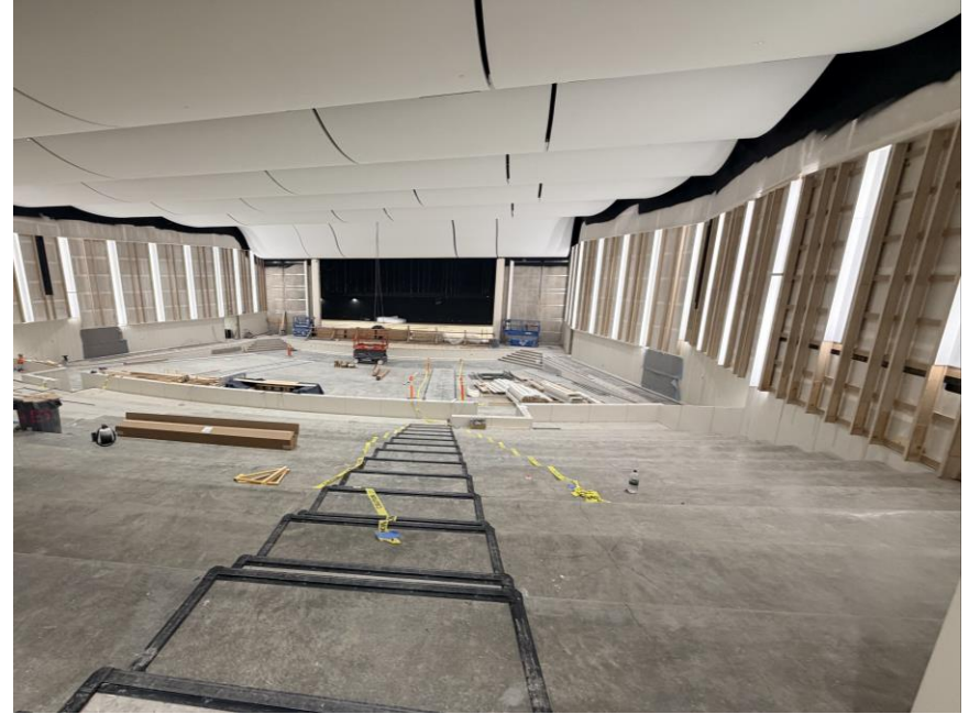
Auditorium aisle lighting installation
