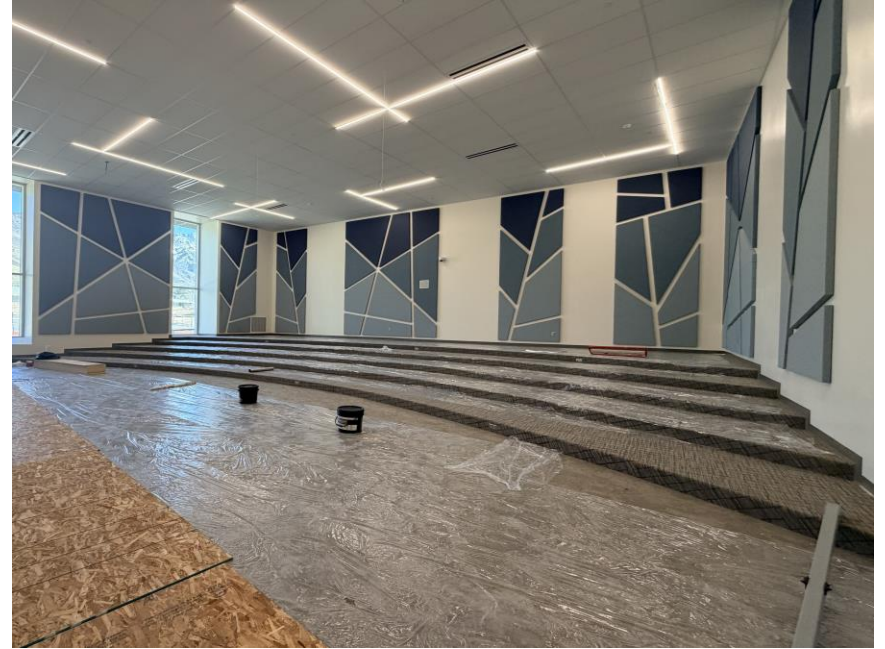
Carpet and acoustical panels installed in the Band & Choir Rooms
