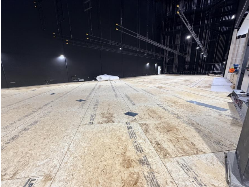
Stage floor installation
