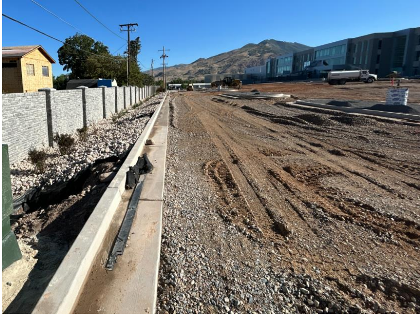
Curb, gutter, landscaping and prepping for asphalt along west property line
