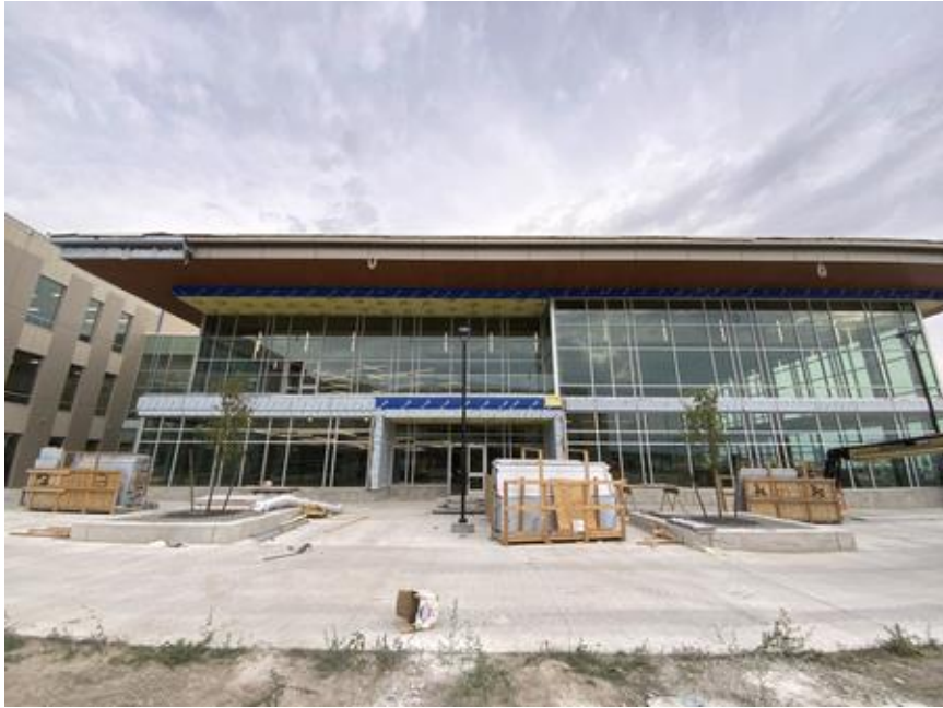
Exterior metal panels outside the Commons
