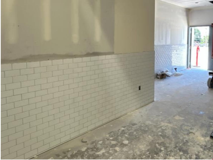
Wainscot tile installation in Corridor
