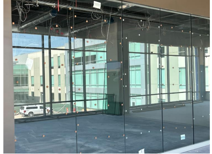
Classroom glazing installed
