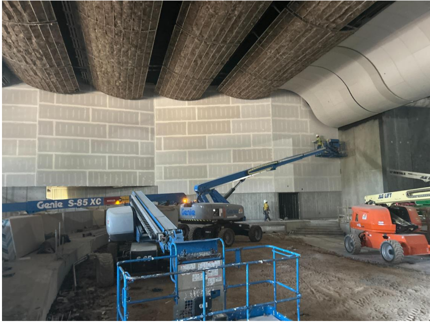
Auditorium ceiling cloud insulation
