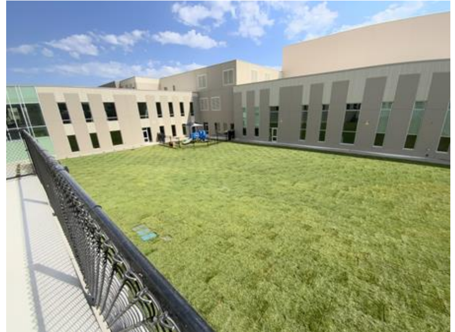
Sod outside the Kindergarten classroom
