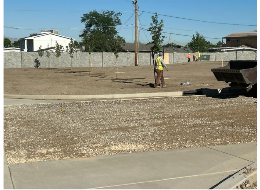
Curb, gutter, landscaping and prepping for asphalt along west property line
