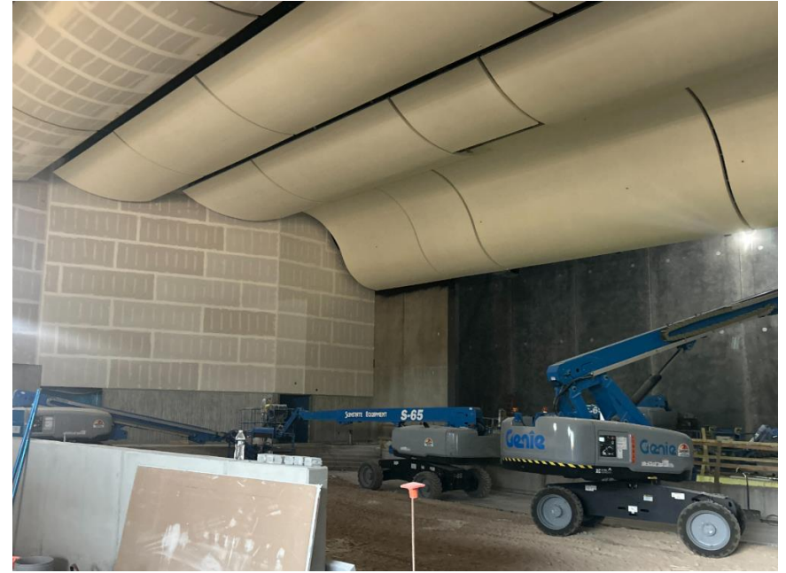
Auditorium ceiling cloud drywall
