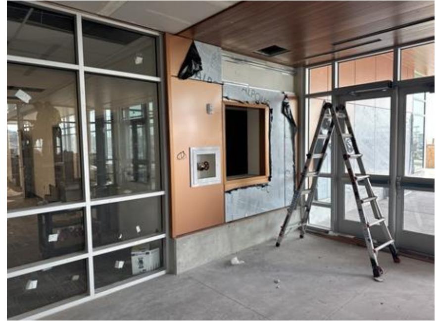
Metal panels in the Main Vestibule
