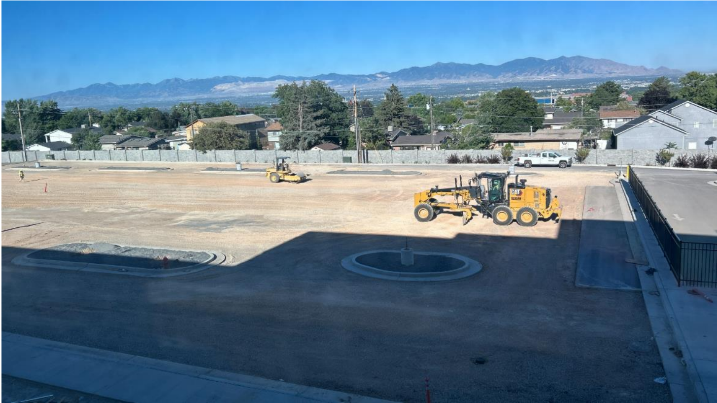
102 West parking lot grading
