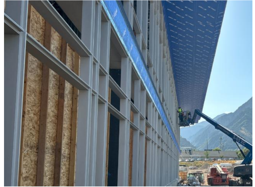
Curtain wall frame installation
