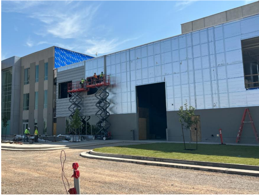
Exterior material installation
