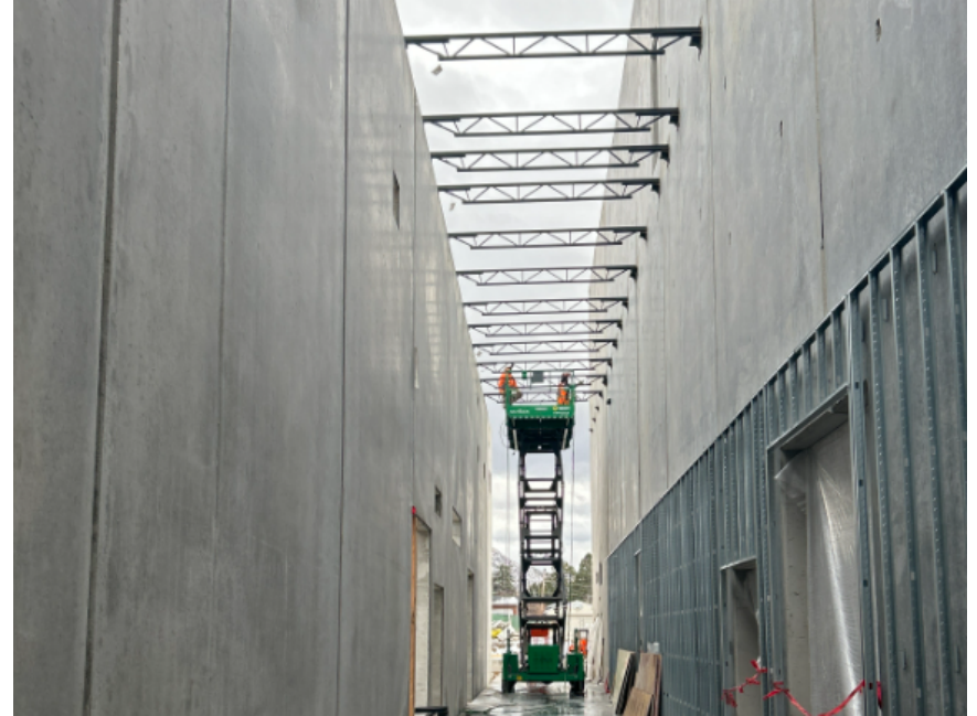
Welding crews installing steel beams and trusses above corridors on both sides of the auditorium
