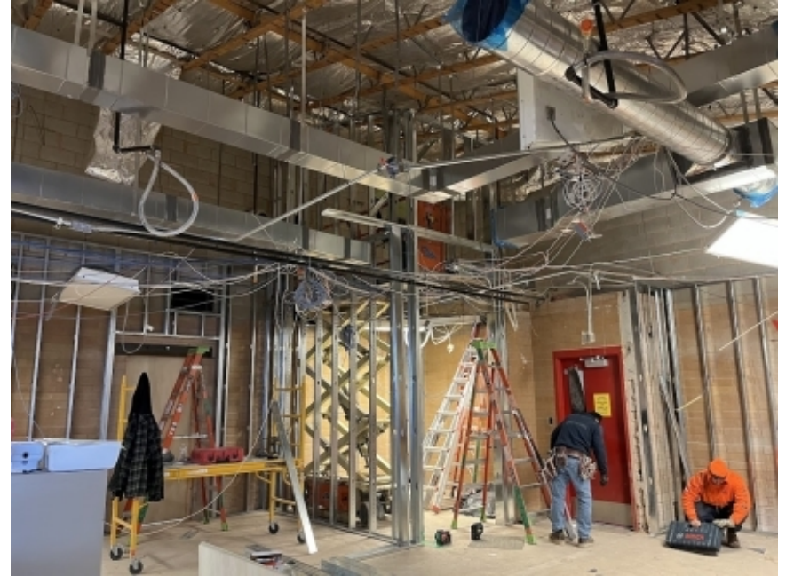
HVAC, ductwork, and framing
