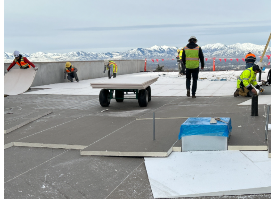
Roof membrane installation
