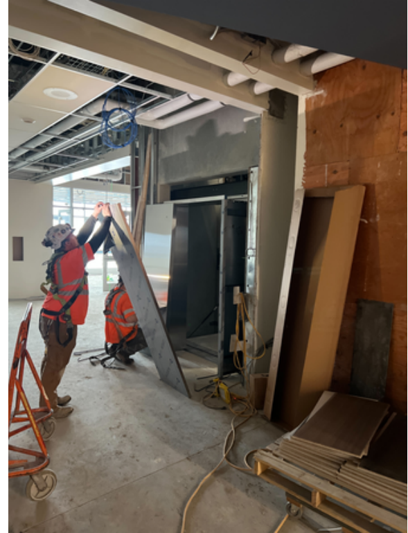
Elevator installation in Performing Arts
