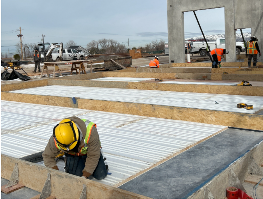
Tilt panel construction
