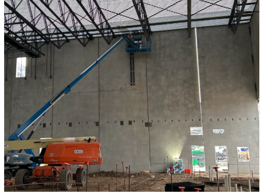
Roof drain installation in two different locations in the Performing Arts phase
