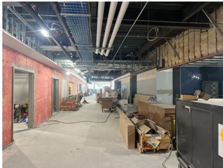
Progress in the Main Entrance
