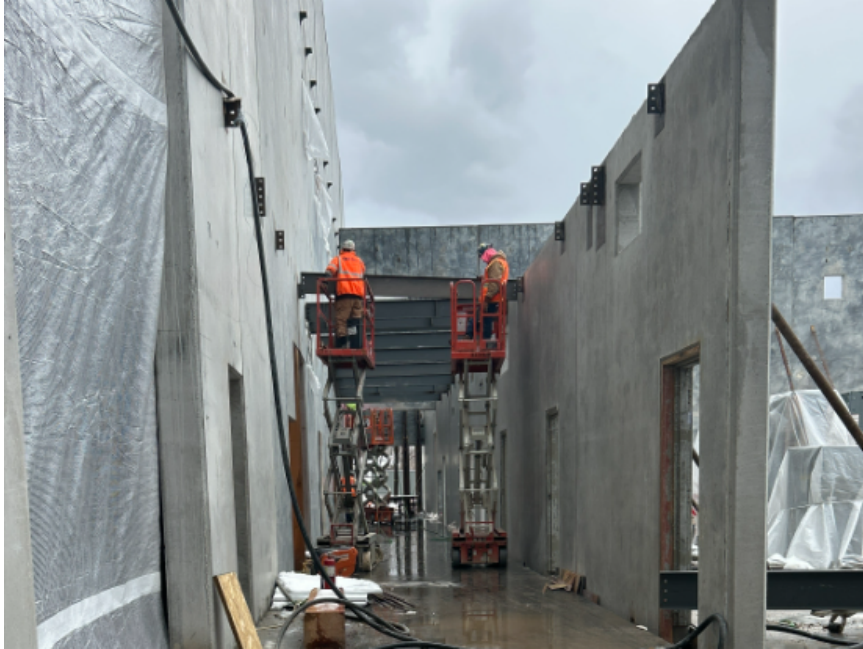
Welding crews installing steel beams and trusses above corridors on both sides of the auditorium
