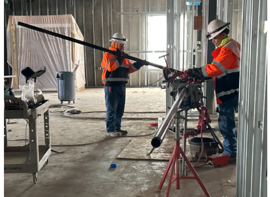
Gas line installation
