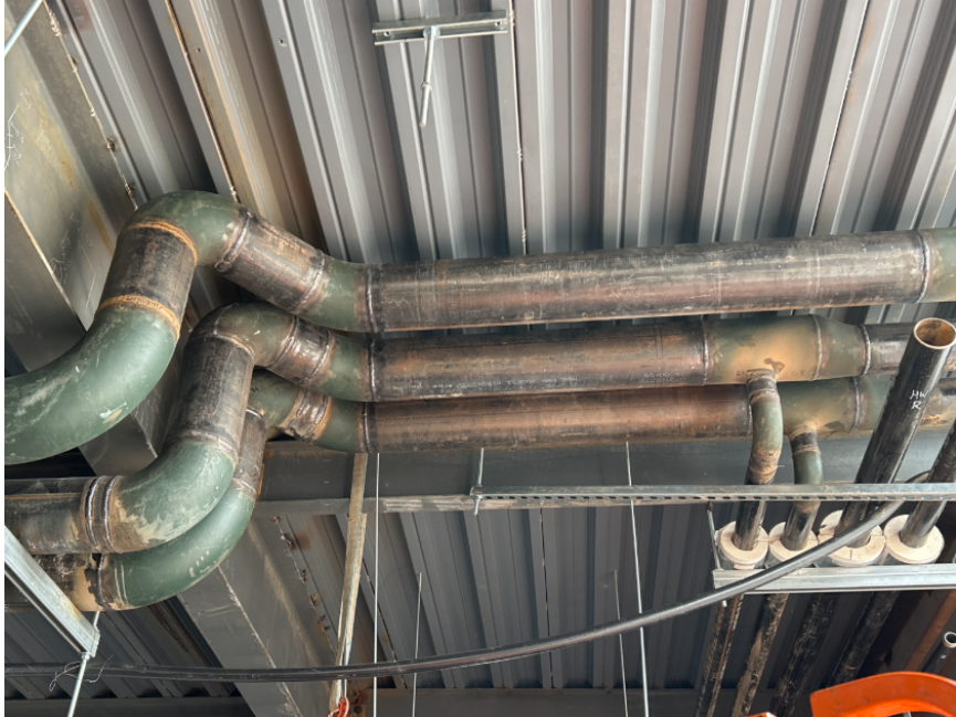
Main water line installation
