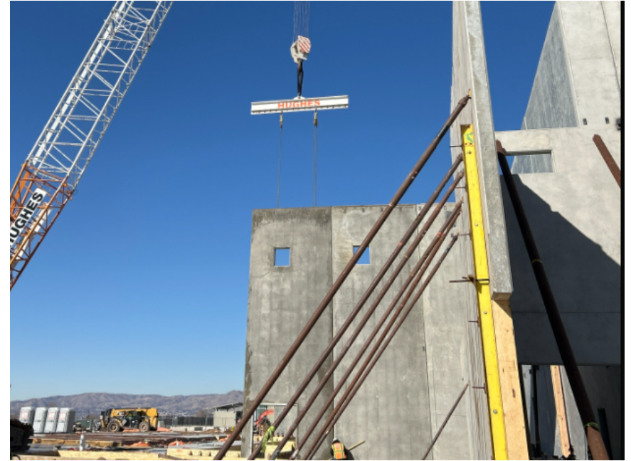
Crews installing tilt panels into place
