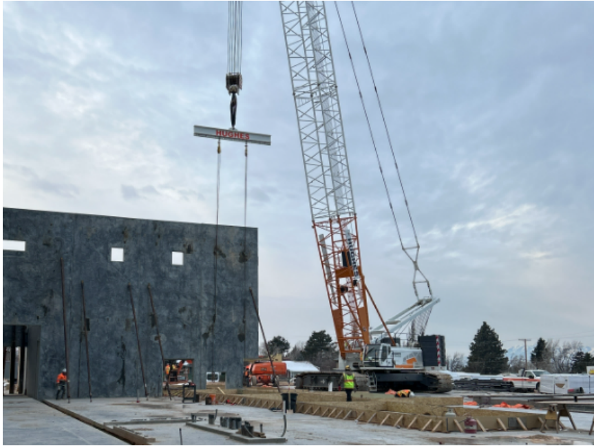
Crews installing tilt panels into place
