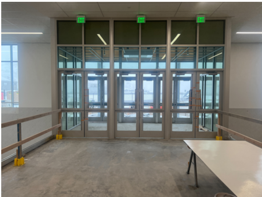
Storefront doors and glass
