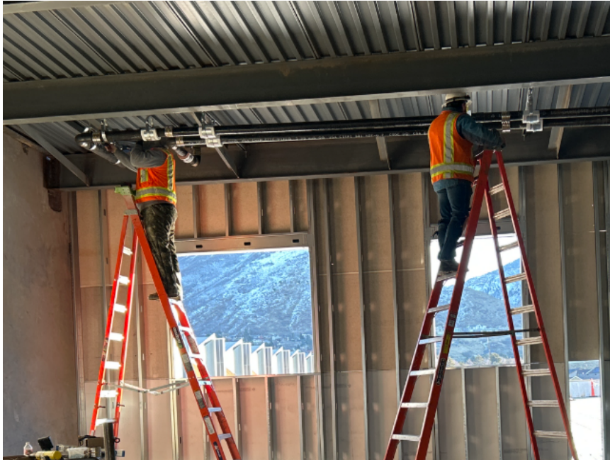
Roof drain installation in two different locations in the Performing Arts phase
