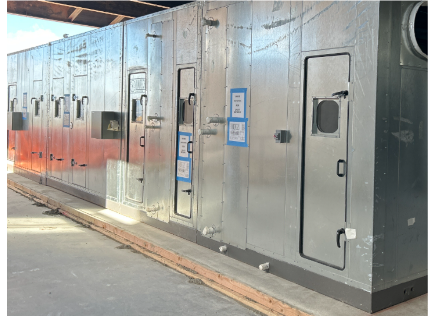
Air handler lifted into place
