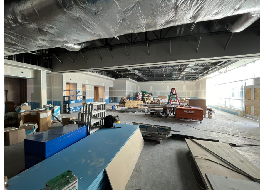
Testing Center with drywall
