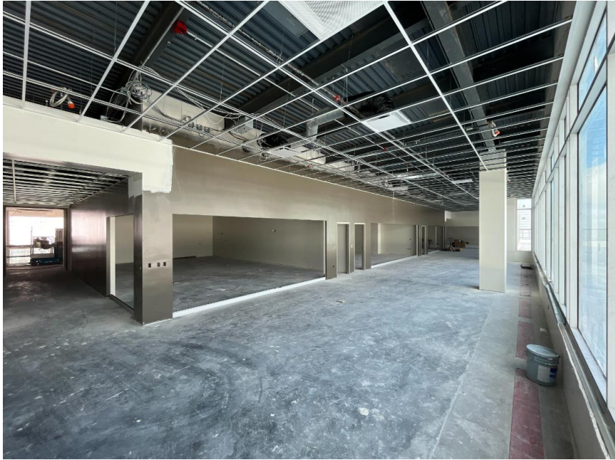
Grid installed and fixed glass walls in progress in Level 3 classroom group 33
