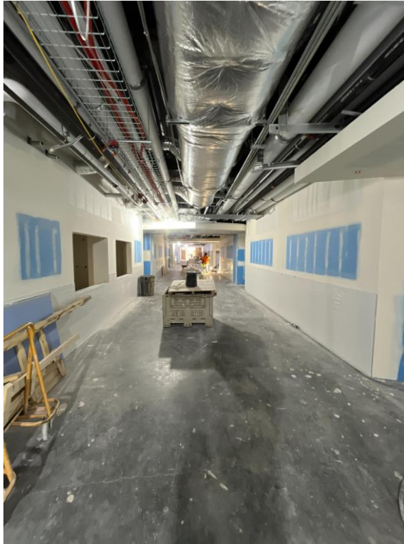
Wall tile in Main Corridor on Level 2
