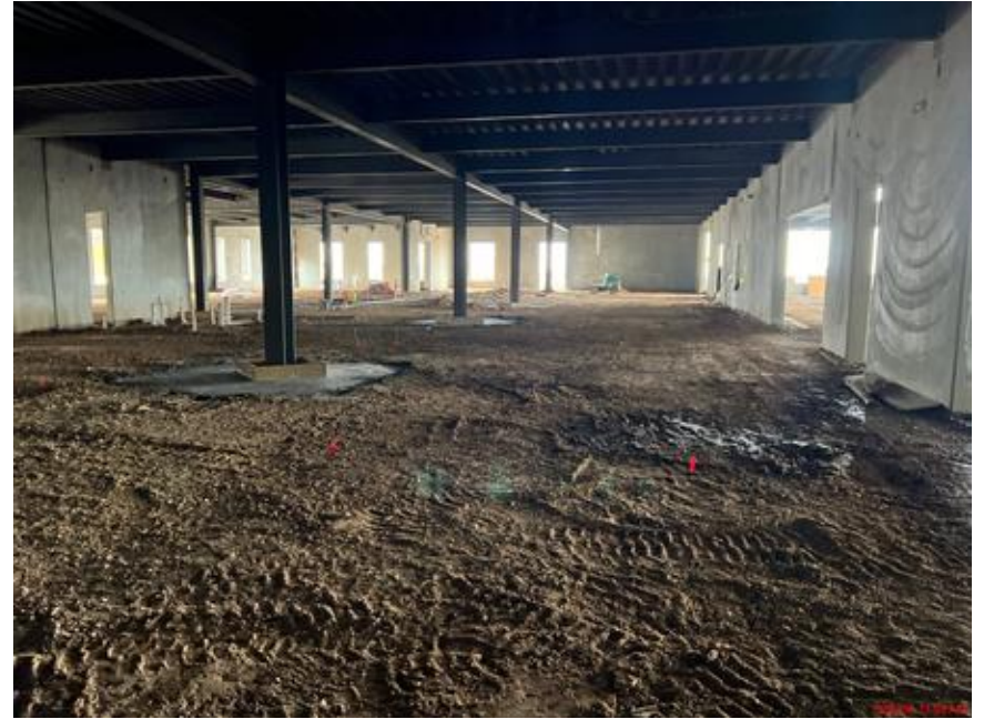
Under slab electrical in the Administrative suite
