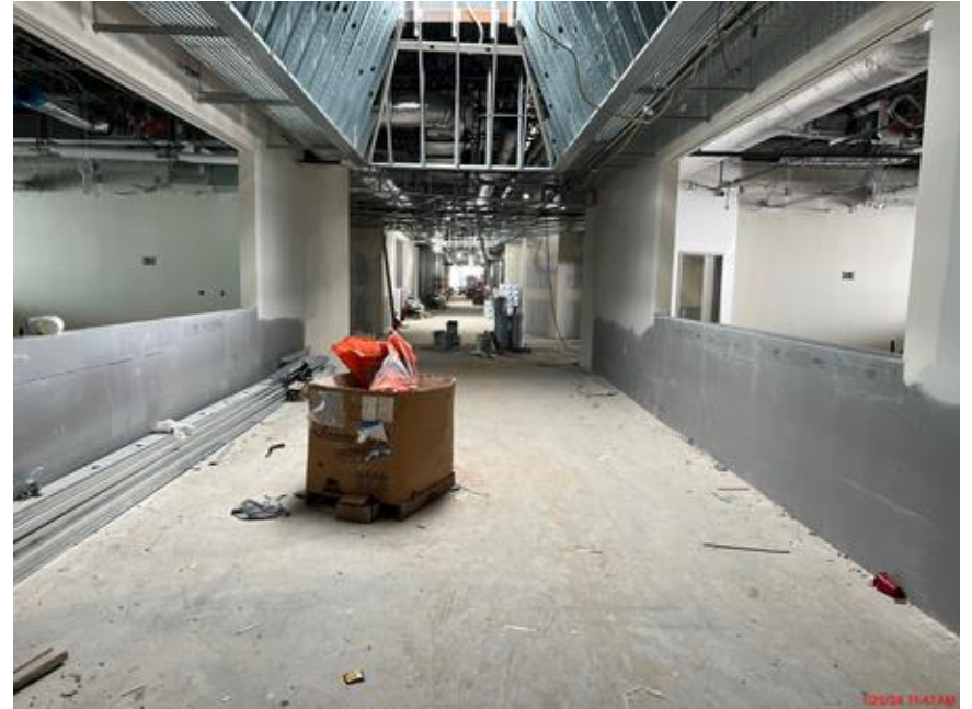
Skylights installed in the Academic building
