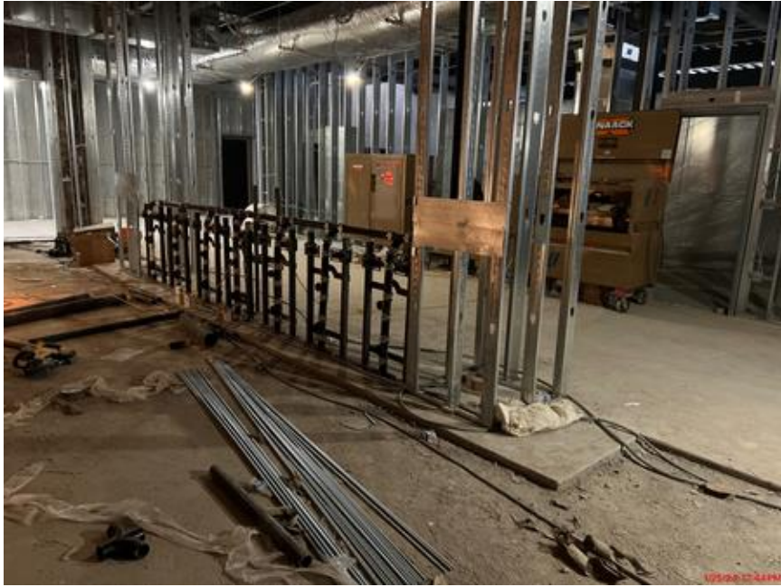
Rough plumbing level 2
