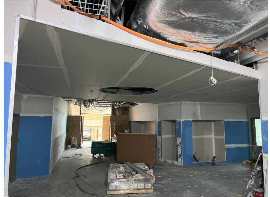
Large soffits outside of classroom groups framed and drywalled
