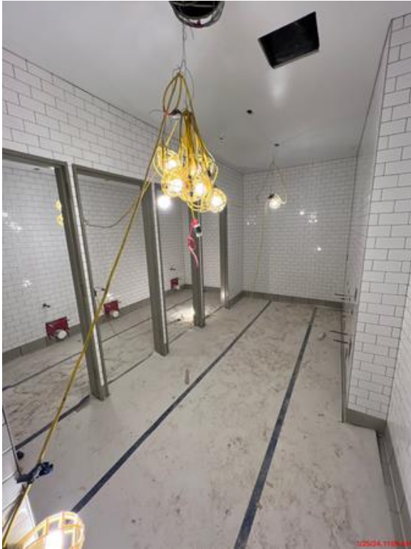
Restroom tile, Athletic building level 1
