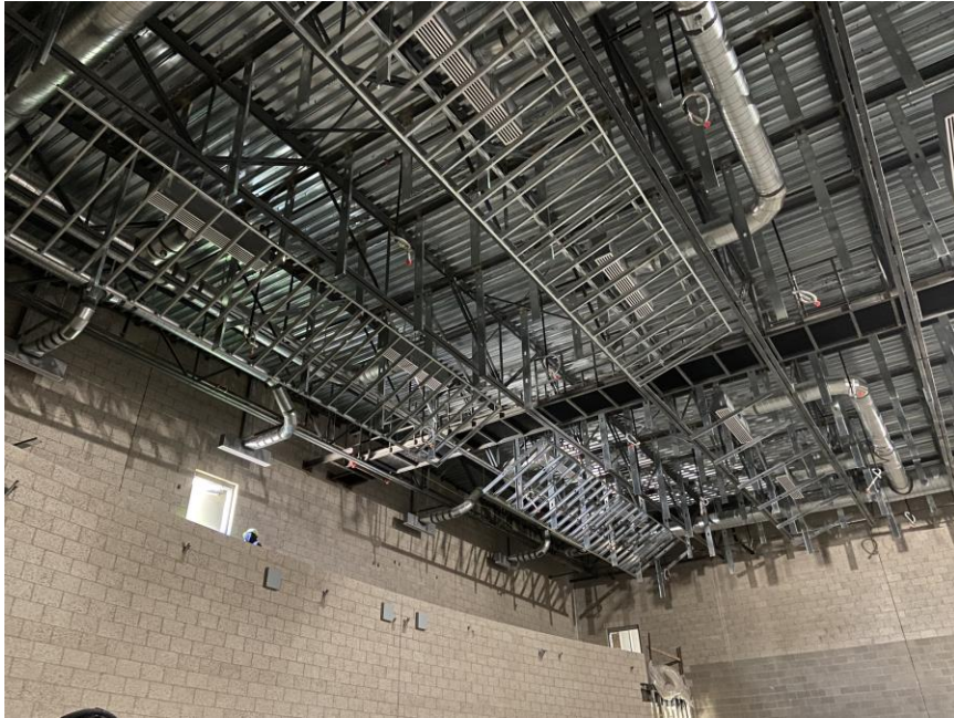
Framing for acoustic sound panels in Auditorium ceiling 17
