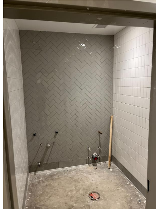
Tile installed in the Administration Suite bathrooms
