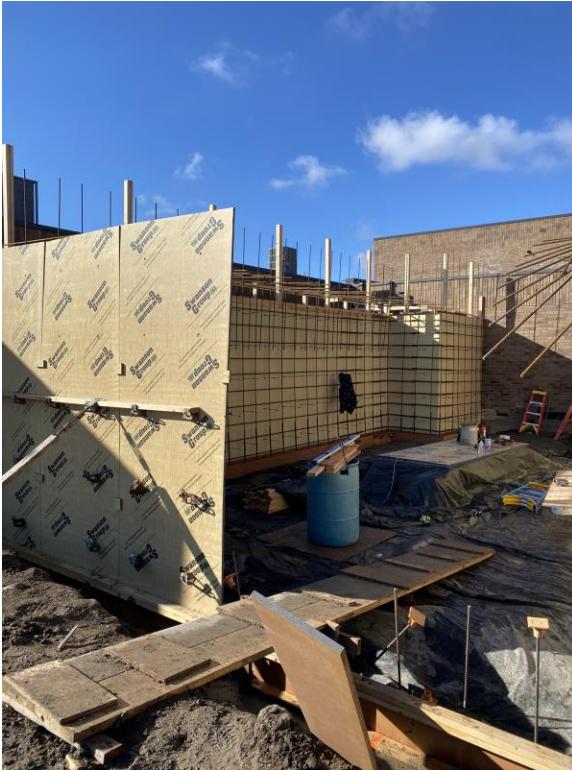
Forms and rebar for the mechanical enclosure
