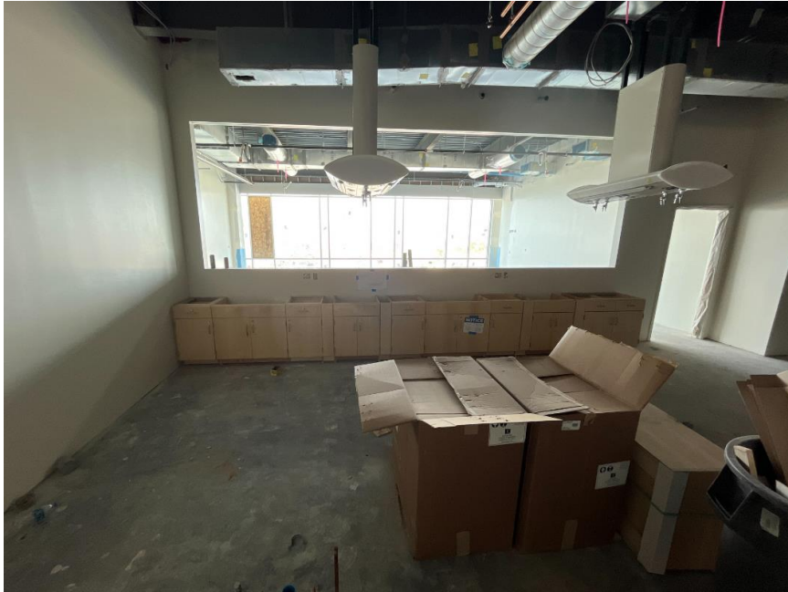
Millwork being installed in the Chemistry Labs on level 3
