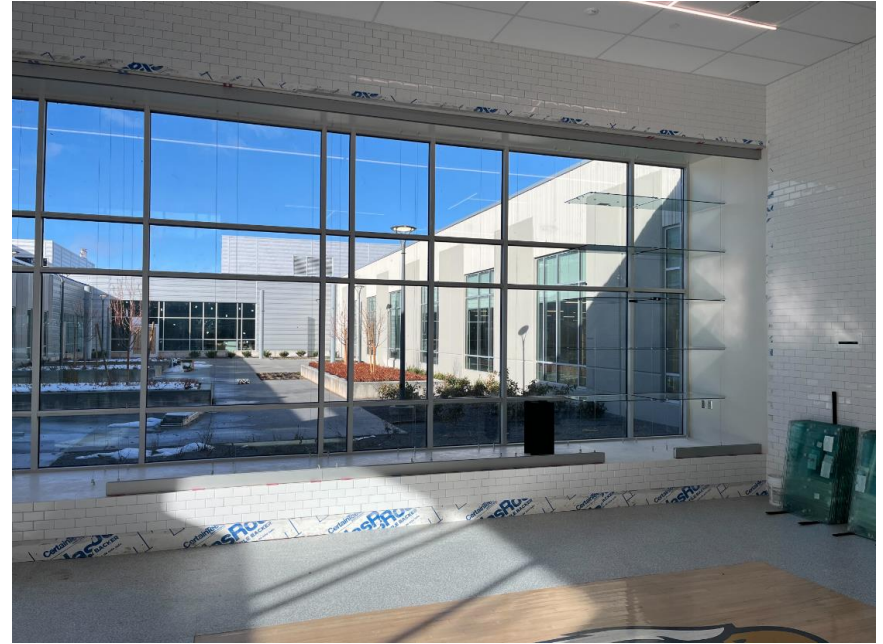
Trophy case glass being installed in Athletics Vestibule
