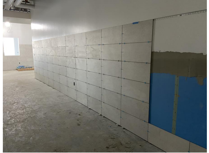
Wall tile work in CTE wing
