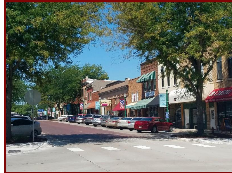
Source: Top is from City of Hickman, Community Center Hickman, NE; bottom is from downtown Ashland, NE
