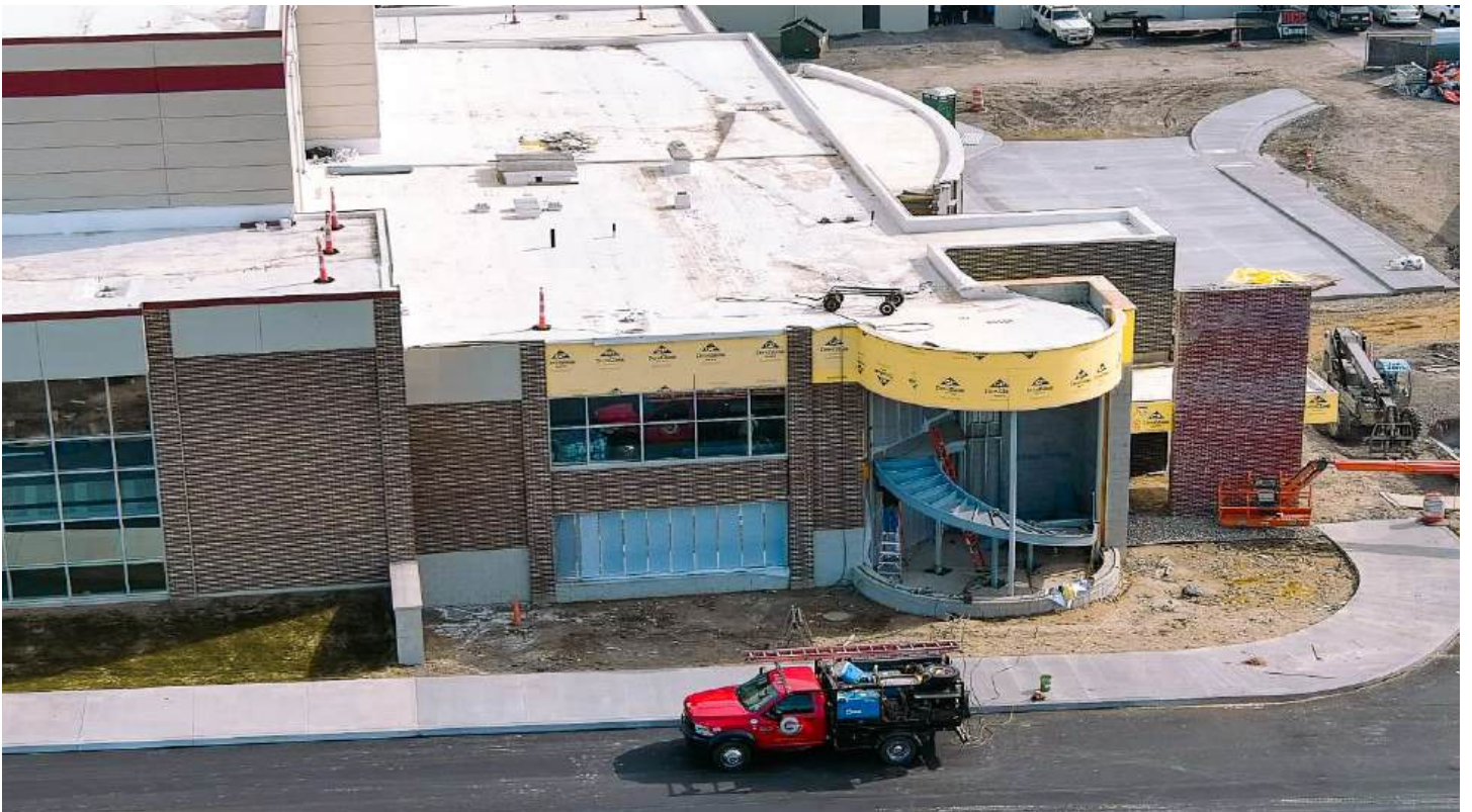
Construction Progress - November 2023
