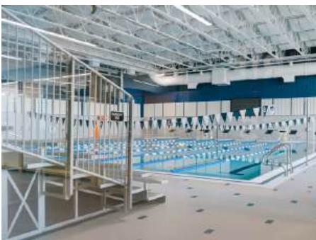
Natatorium with a 25 yard, 8 lane pool.
