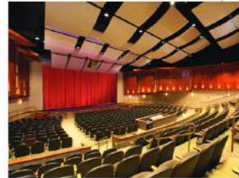
Acoustical panels similar to those in a theater designed by Shuler Shook will be added in the Yizhuang theater during the next phase of design.
