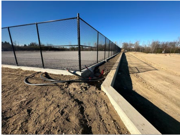
Field Retaining Walls
