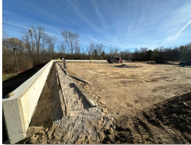
Concrete Retaining Walls
