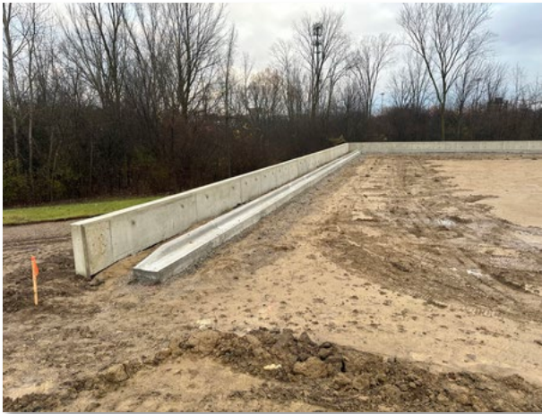
Parking Retaining Wall
