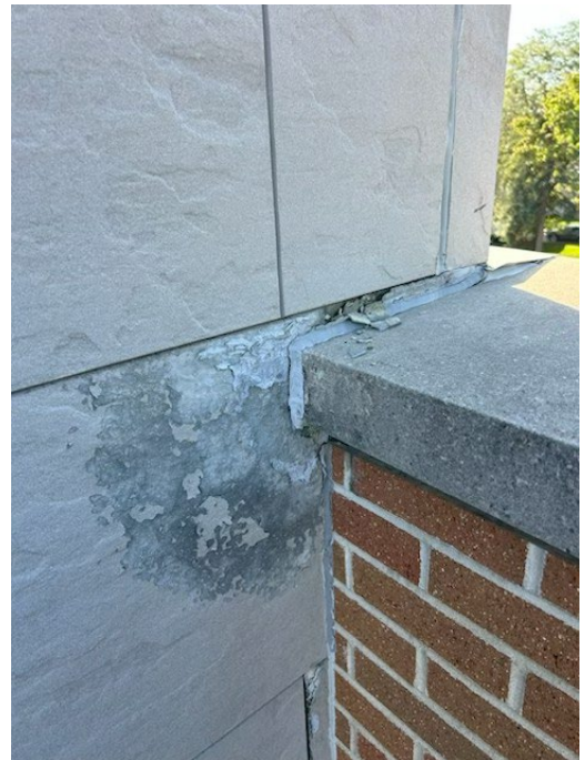
Resealed exterior wall joint
