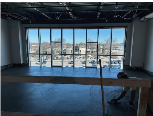
Concrete for offices being smoothed.
