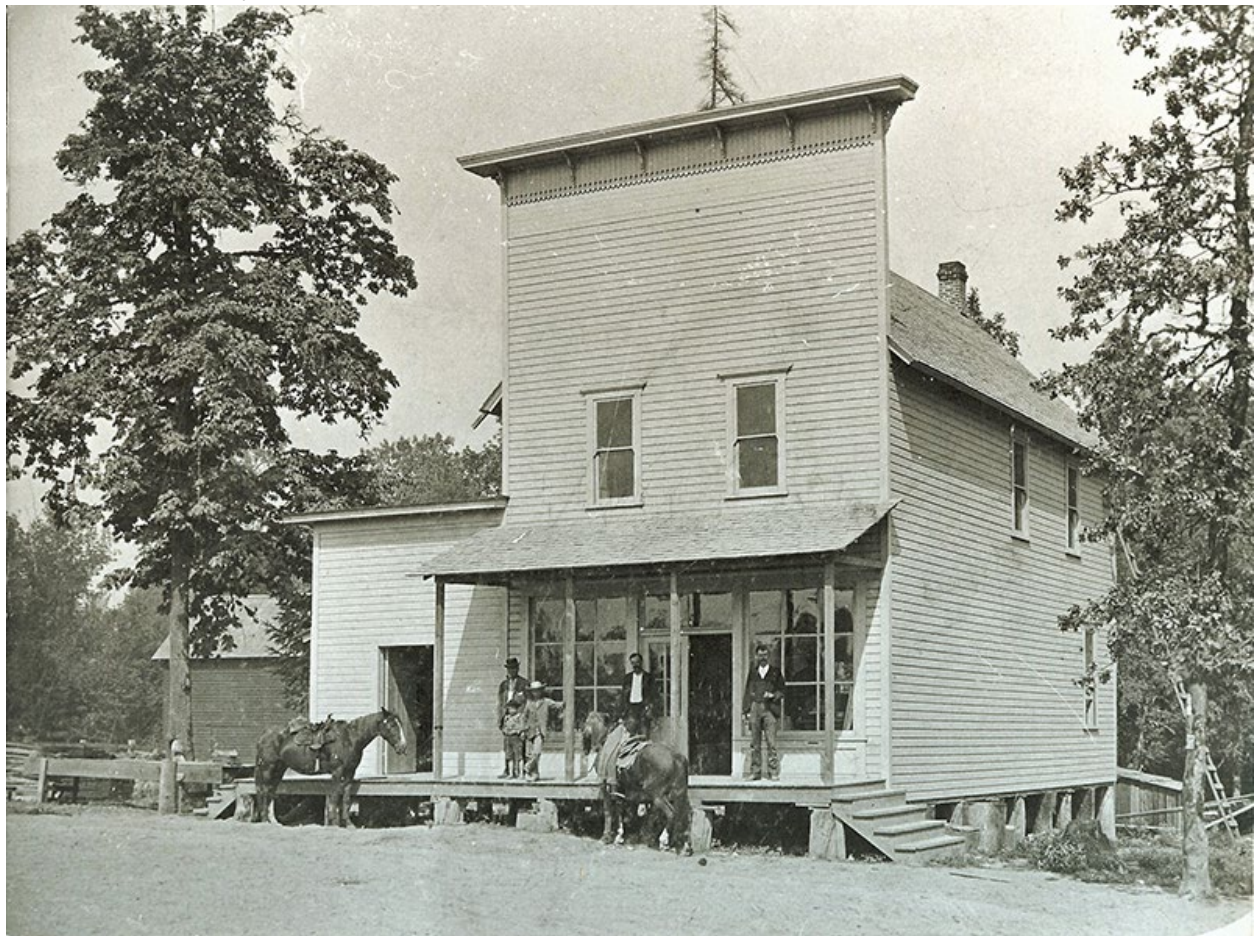
First Store in Banks, built about 1901 on North Main Street near Banks Rd.
