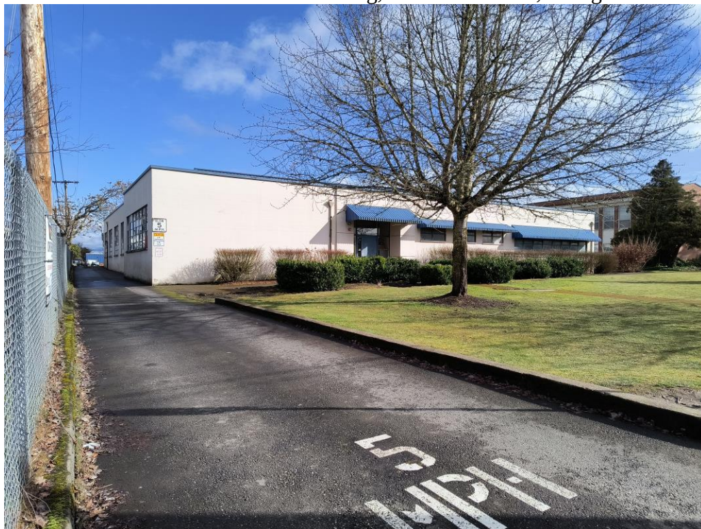
Exterior view of 1951 Vocational building, northwest corner, facing southeast.
