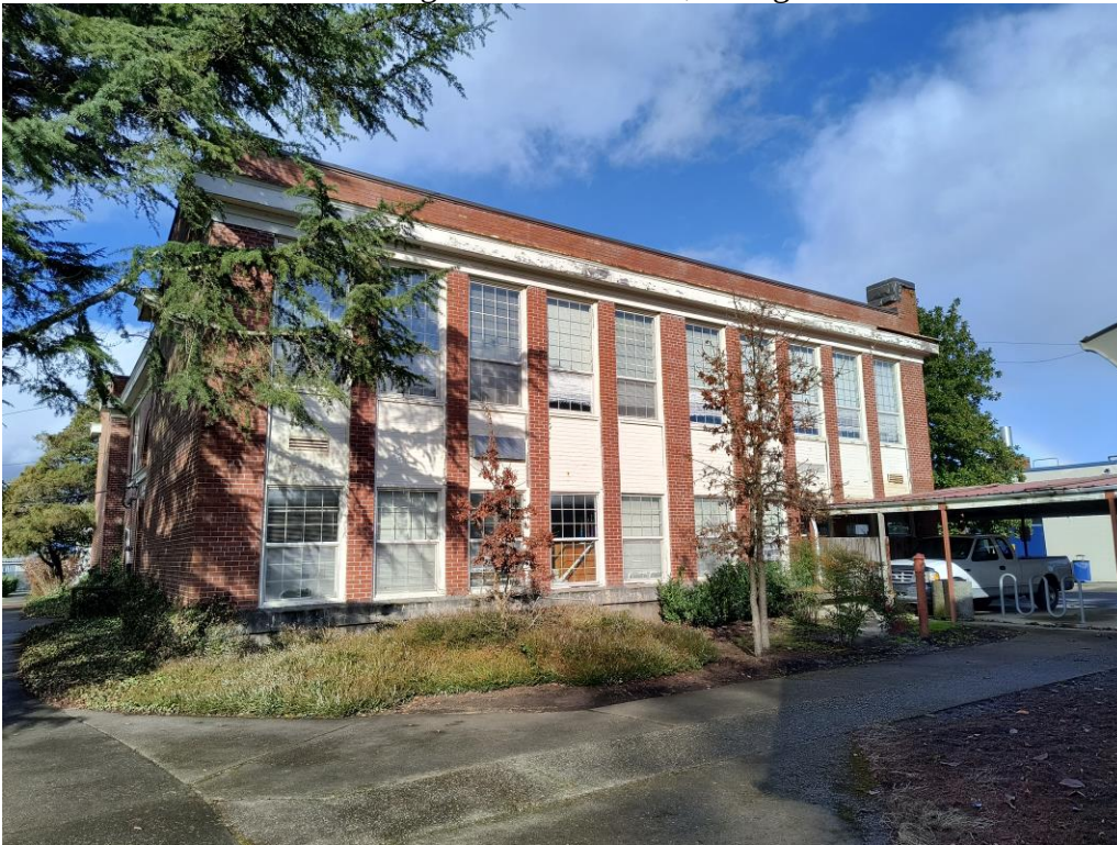
Exterior view of the southwest corner of the 1920 building, facing northeast.
