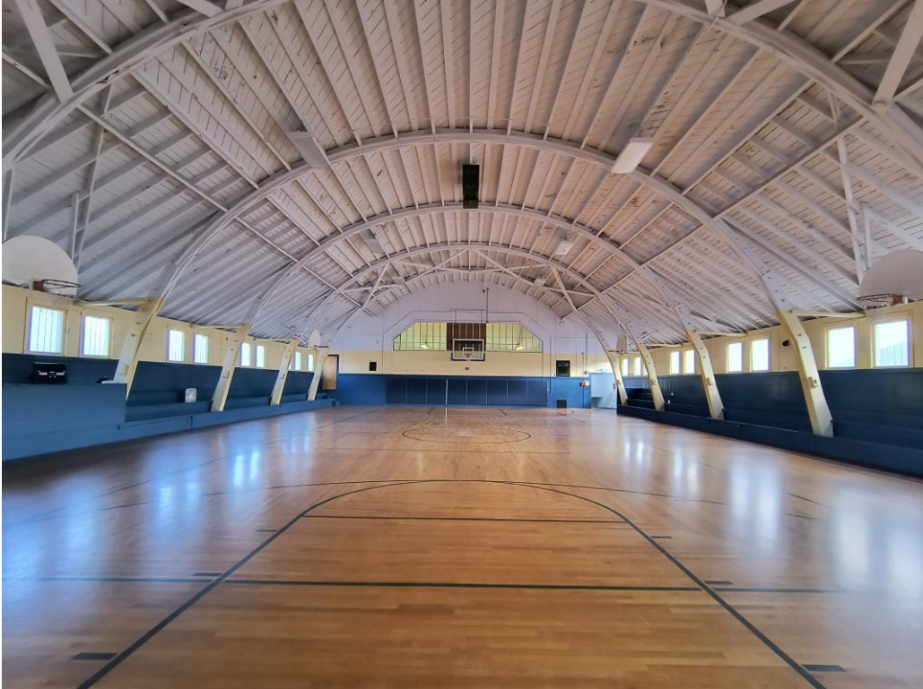
Interior view of 1936 building, west side, facing east.
