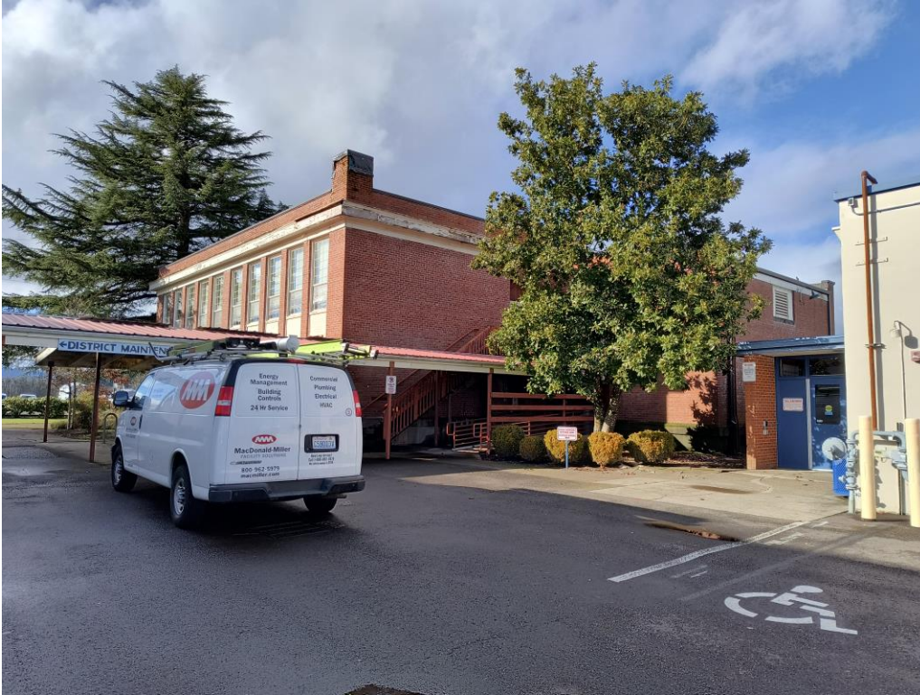
Exterior view of 1920 building southeast corner, facing northwest.
