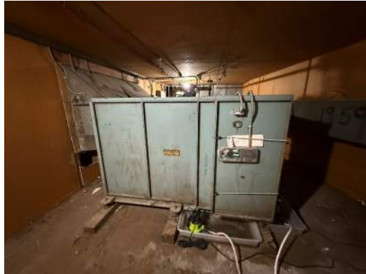
Figure 6 The gym air handling unit has steam heating coils and while currently functional, is past end of useful life.
