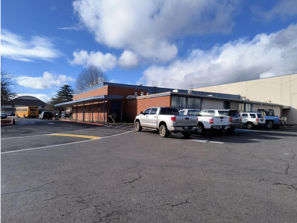
Exterior view of 1959 building, southeast corner of cafeteria area, facing northwest.
