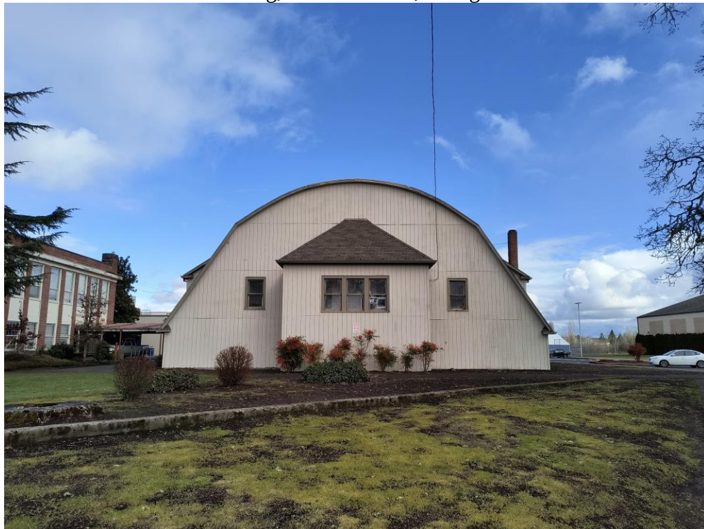
Exterior view of 1936 building, west elevation, facing east.
