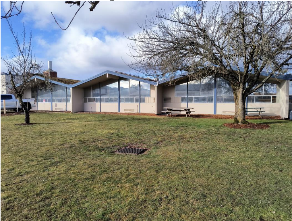
Exterior view of 1959 building, south elevation, facing north.
