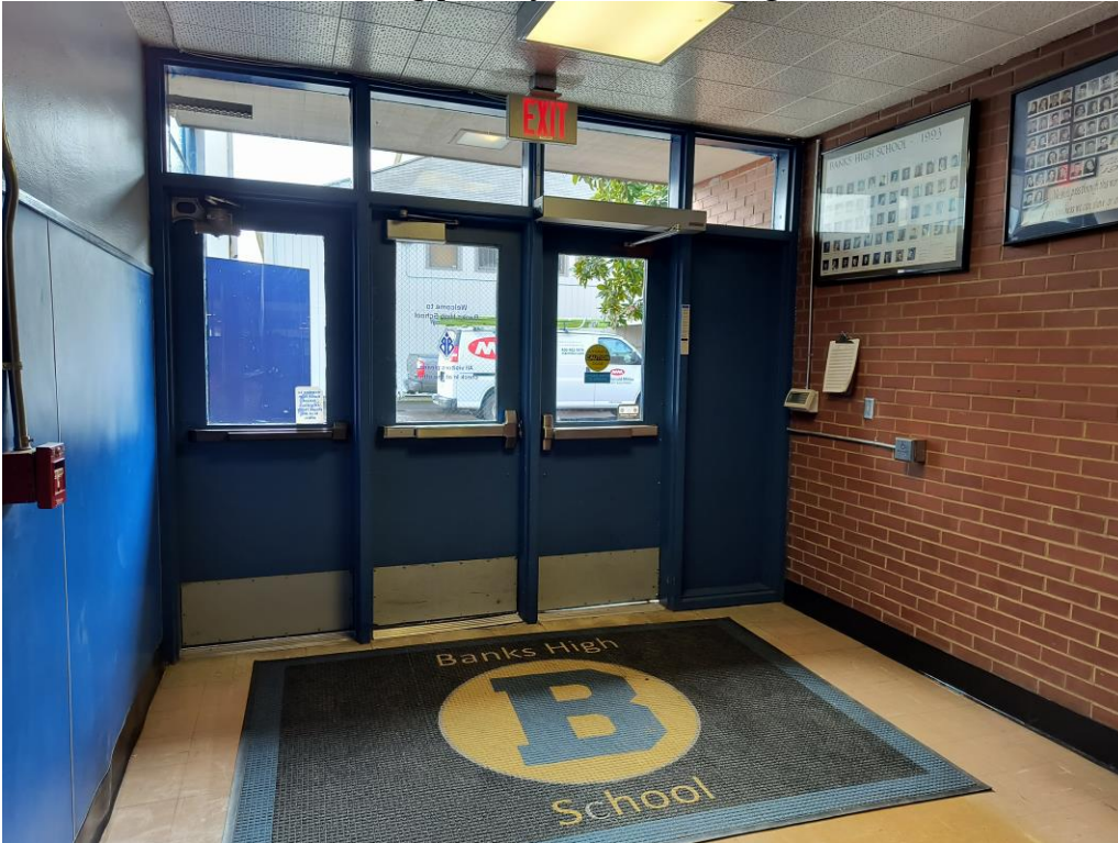
Interior view of 1959 building primary entrance, facing south.
