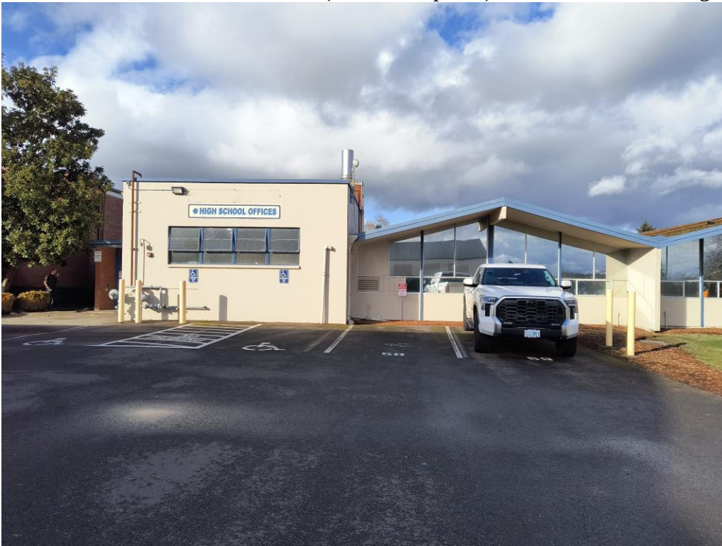
Exterior view of 1951 Boiler room (left side of photo), south elevation, facing north.
