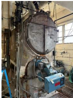
Figure 5 The existing steam boiler is aging and minimally functional. Steam distribution throughout the building is failing and sections of piping have had to be valved off to prevent leaks coming up through flooring.
