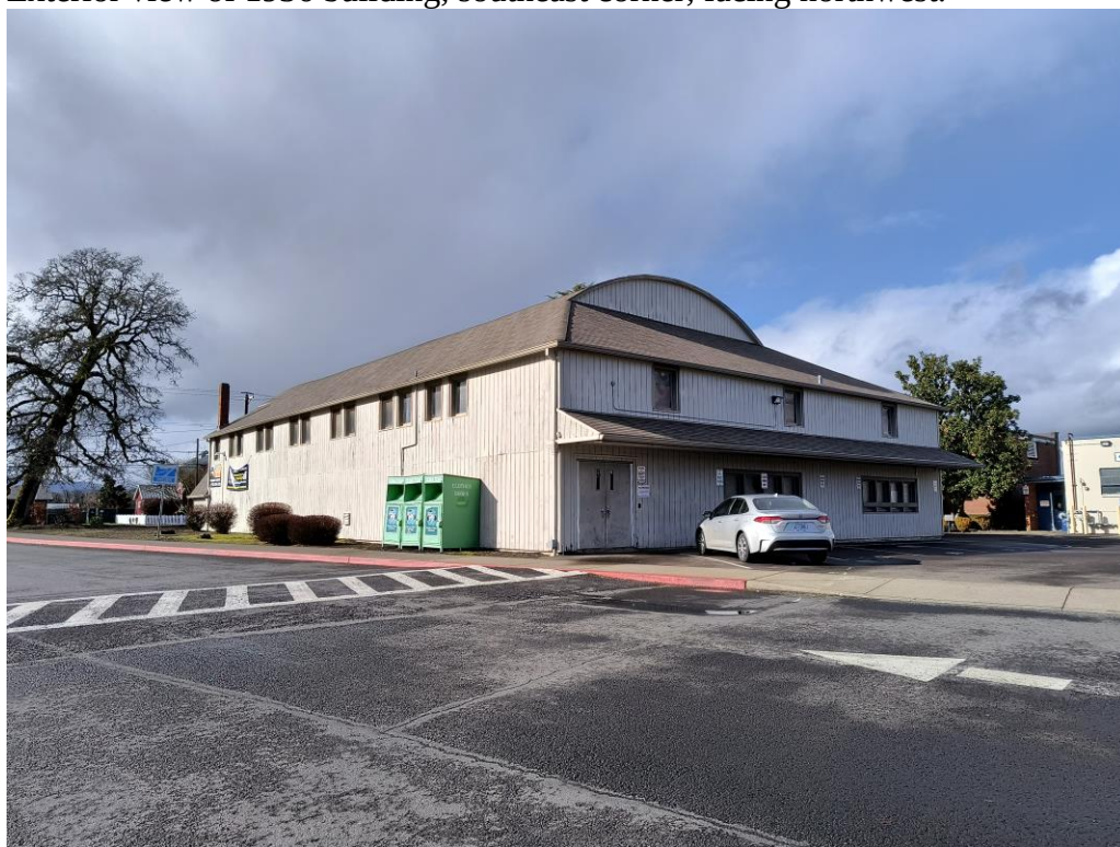
Exterior view of 1936 building, southeast corner, facing northwest.
