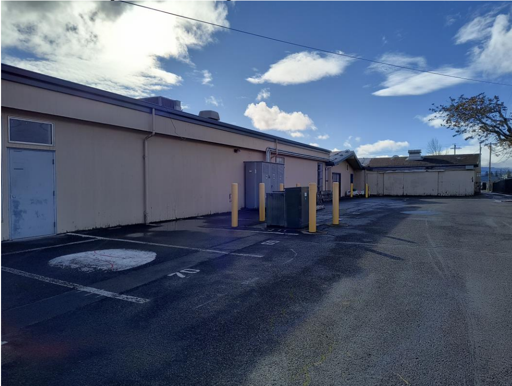
Exterior view of post-1959 building, western northeast corner and north elevation, facing southwest.
