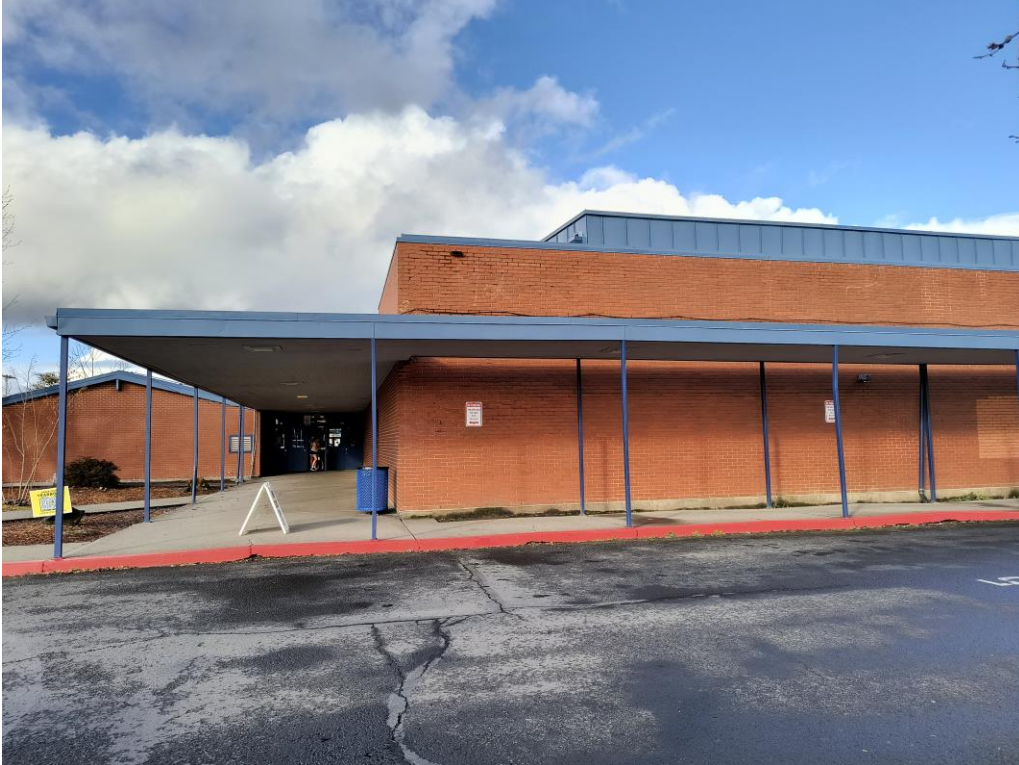
Exterior view of 1959 building, southwest corner of cafeteria area, facing north.
