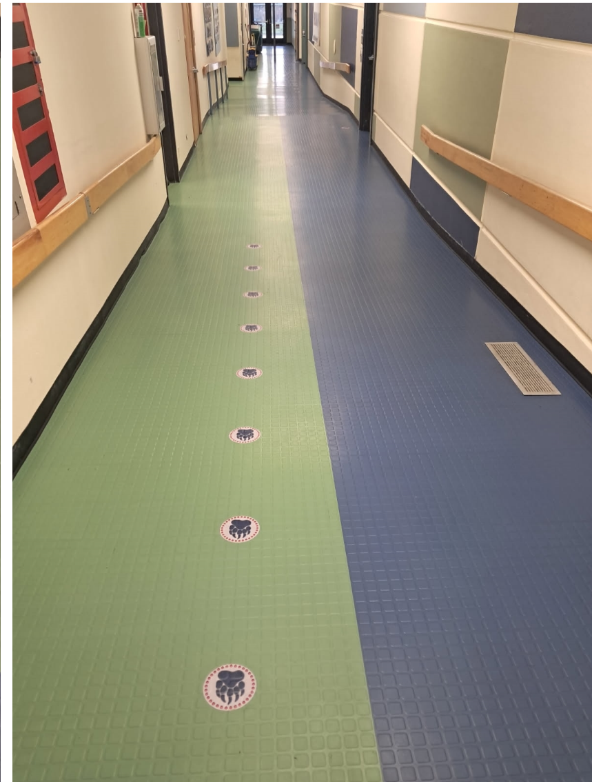
Y.V. Finished non-slip floor
