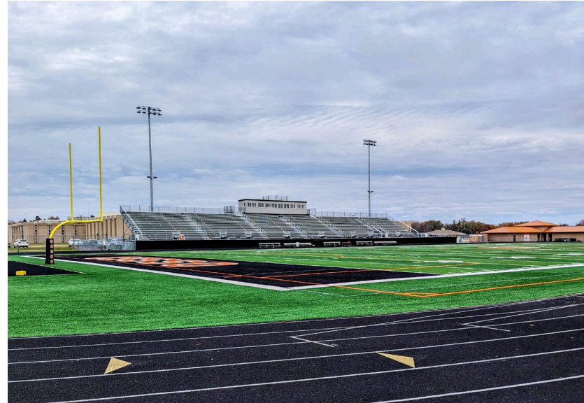
Power, Lights, Bleachers, and Turf
