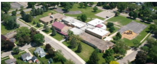
BANFIELD ELEMENTARY SCHOOL 301 17th St NW 507-460-1200
