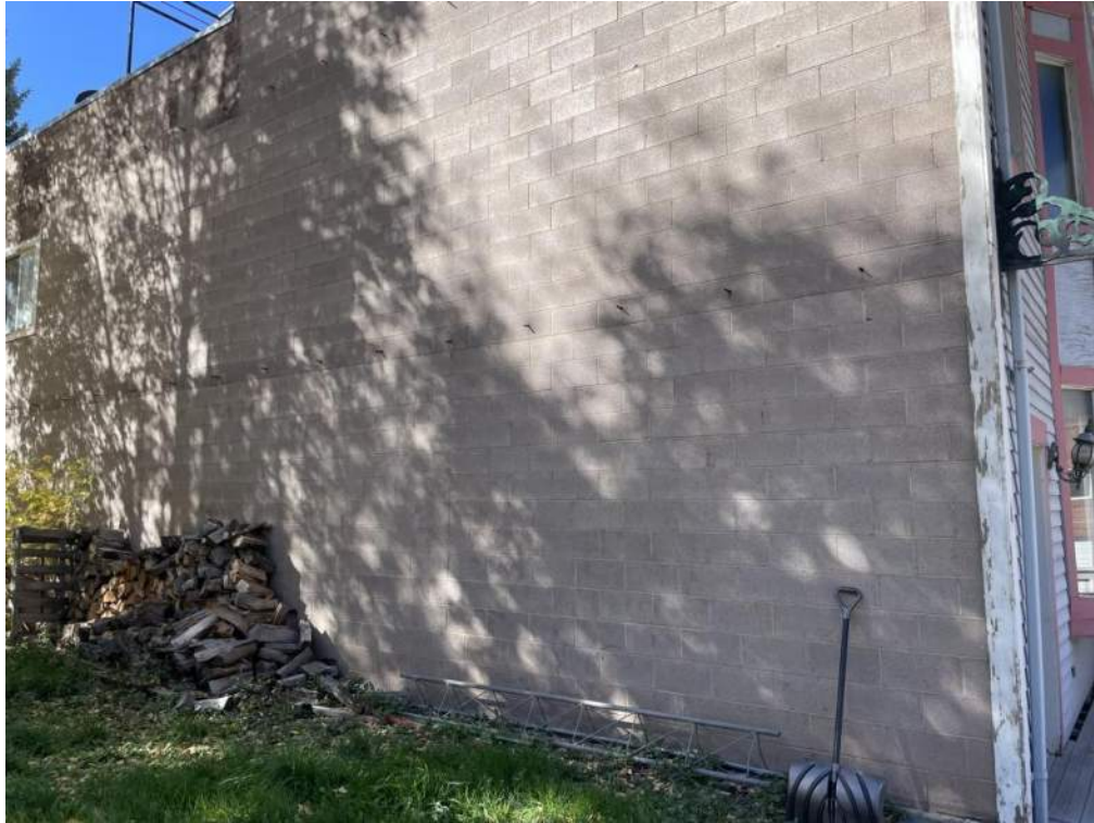
Figure 11- Exterior load-bearing CMU wall.
